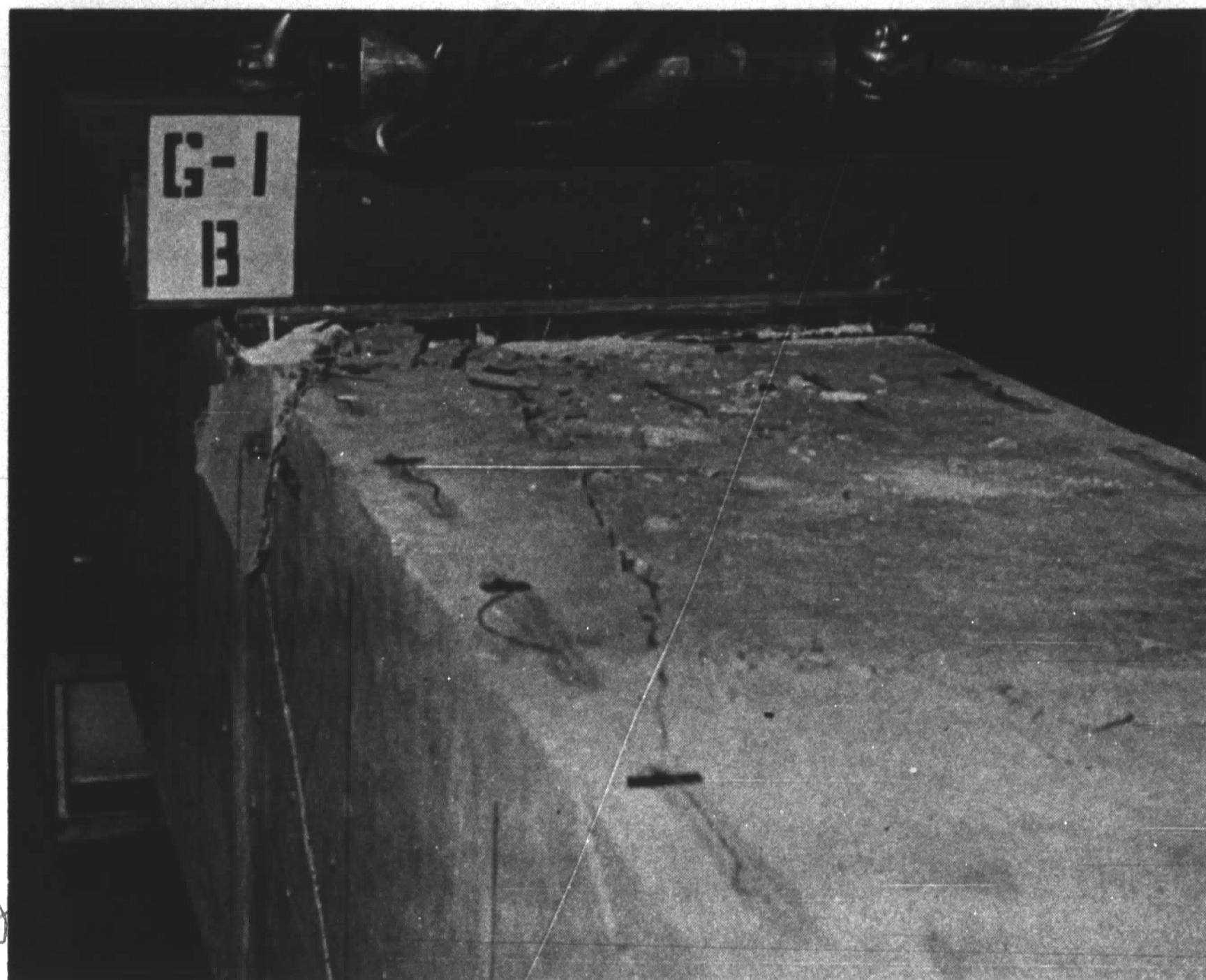
d. Left Side and Top Flange of B Load Point After Failure
