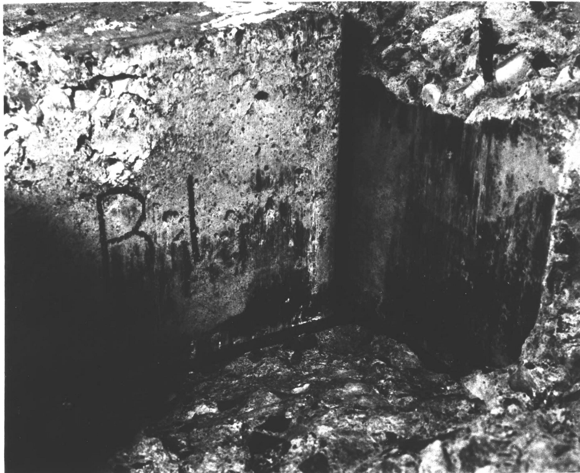
Fig. 18 CONCRETE AT EXTERIOR CORNER AFTER REMOVAL OF PILE - TEST 2
