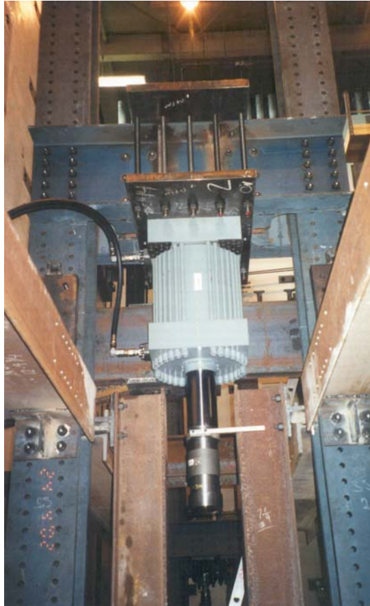
(a) Frame FR2 during construction
