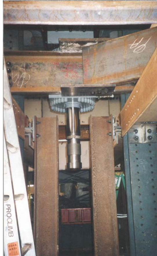
(b) Frame FR2 after construction
