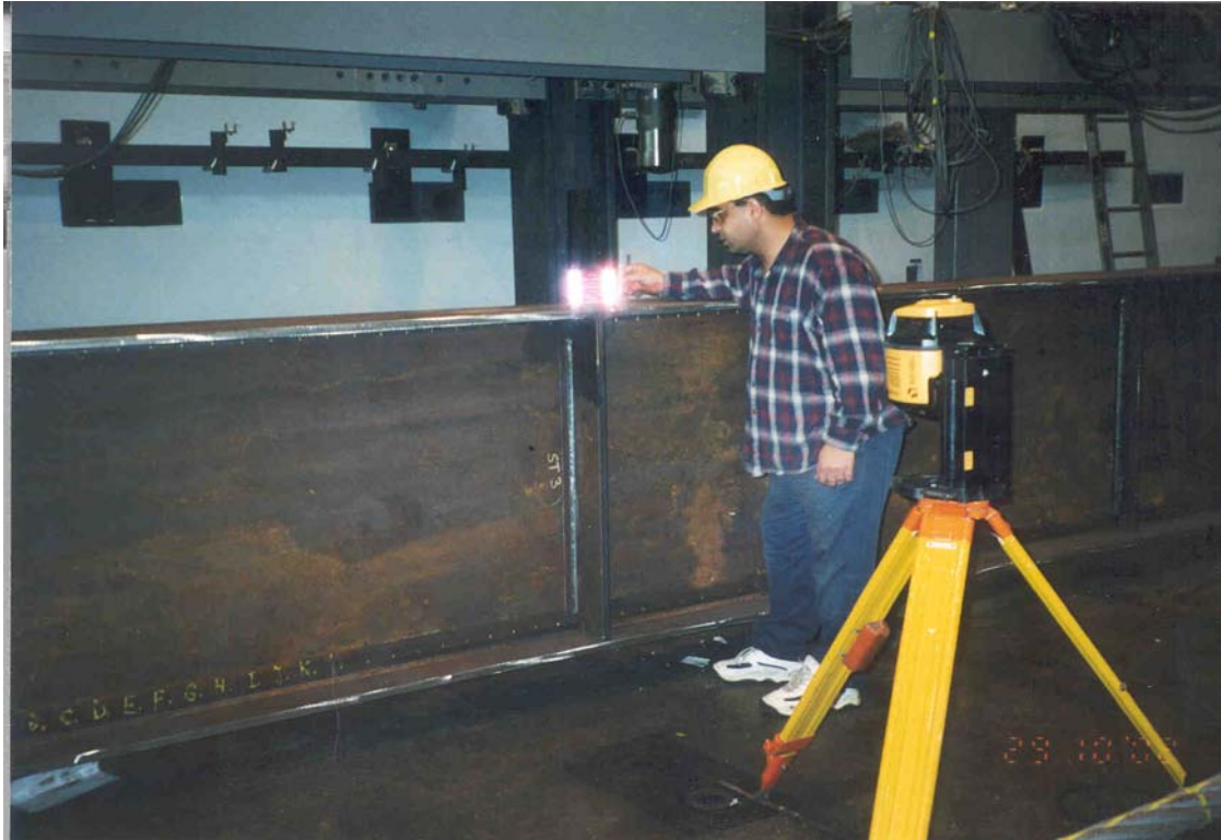
Figure 4.28 Flange imperfection measurements using 1485HP laser level
