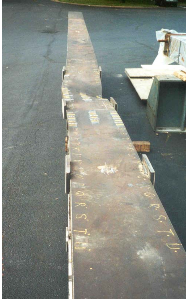
Figure 5.137 Lateral distortion of compression flange (Specimen 7)
