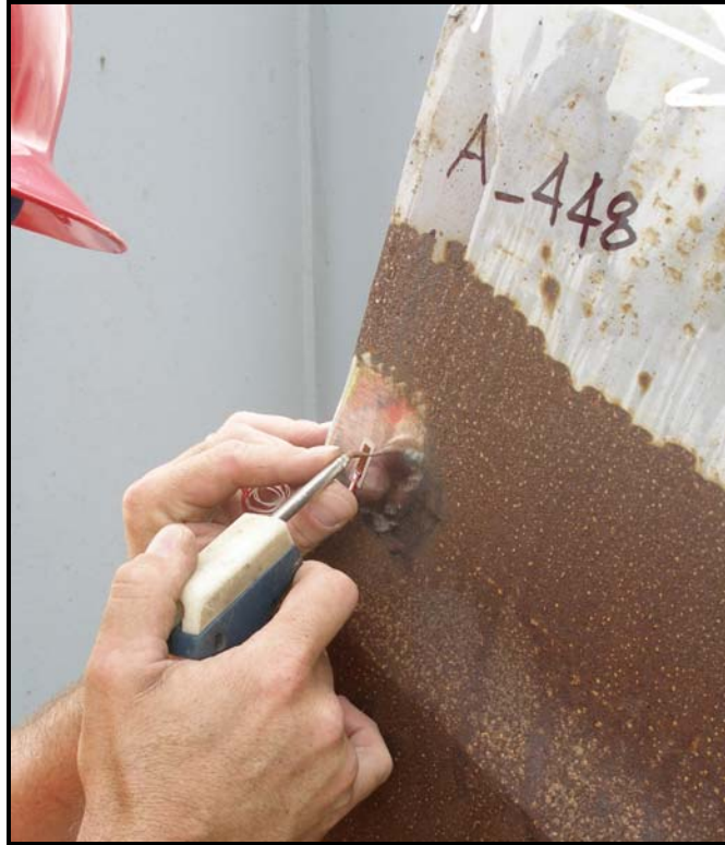
Figure 2.1 – Installation of weldable strain gage adjacent to Weld A_448
