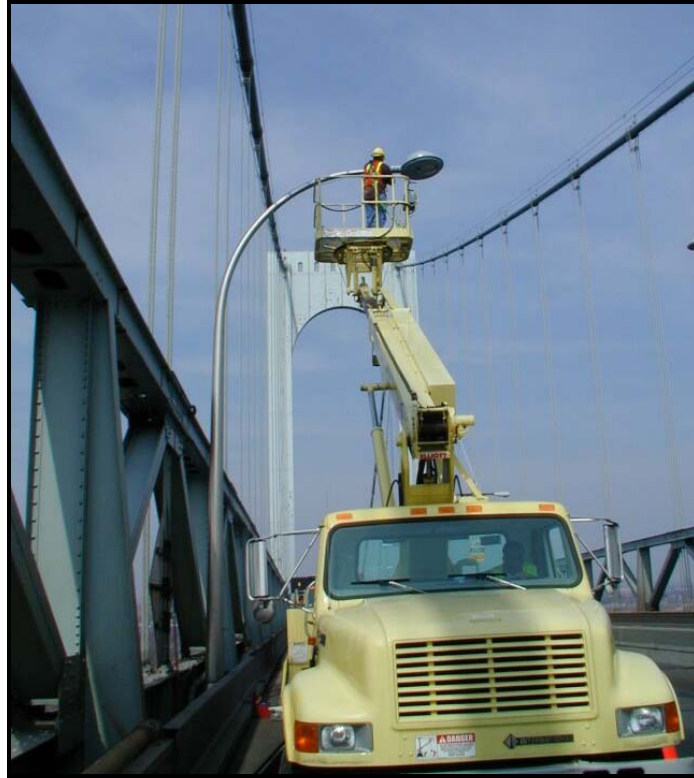
Figure 3.3 – Prototype light pole located on the Bronx-Whitestone Bridge
