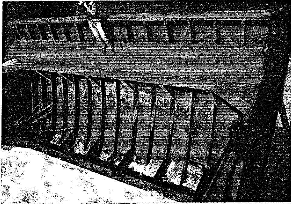
Figure 15: Tainter Gate at Lock & Dam #5 (6/92/5-7)
