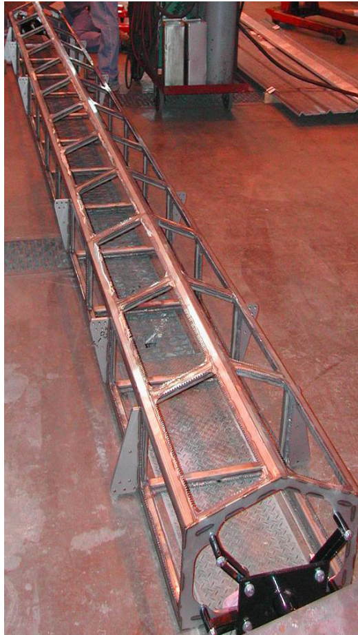
Fig. 3. Finished AL-6XN stainless steel truss before sandwich panels were mounted. Load-introduction brackets are on the sides of the girder.
