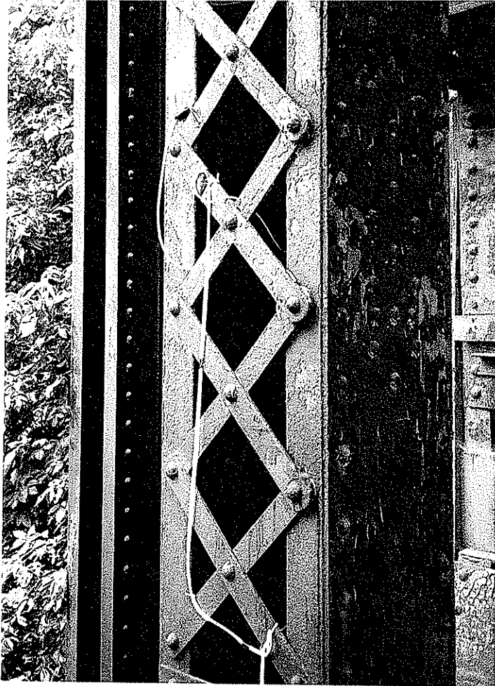
(a) Gage 27.98 at SW corner of post (8/98/9-3)
