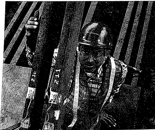
Left: Top View of Group of 8 Lower-Chord Eyebars (8/98/7-5) (Diagonal eyebars L5U6 in foreground)
