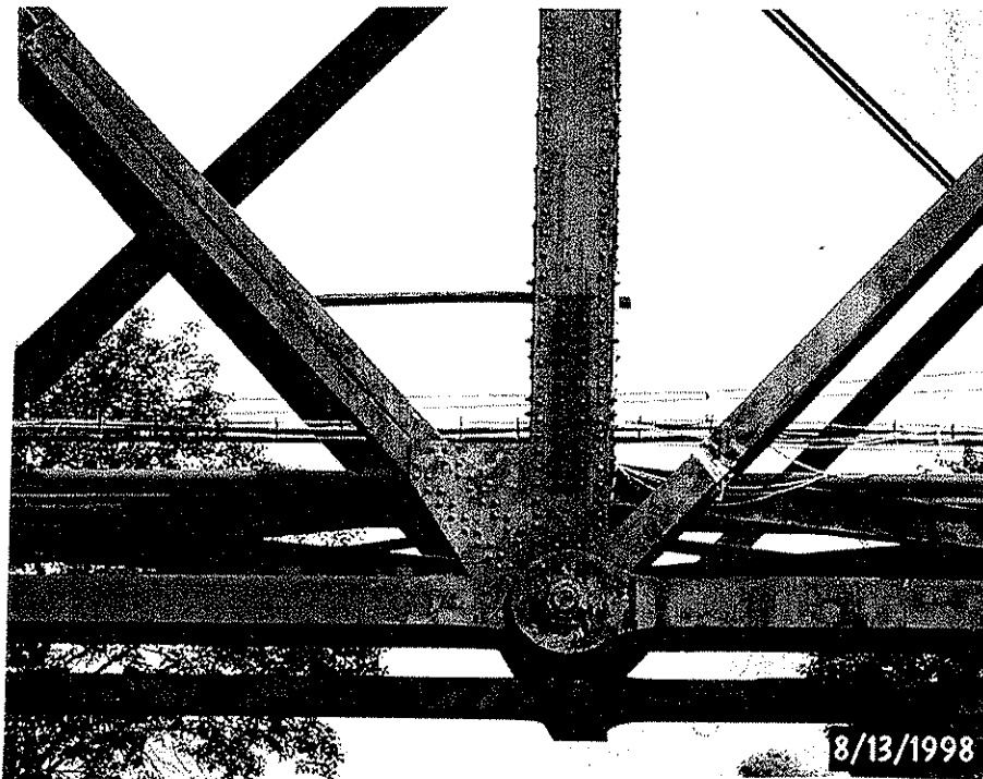
(b) East side of Post L5U5-East after retrofit
