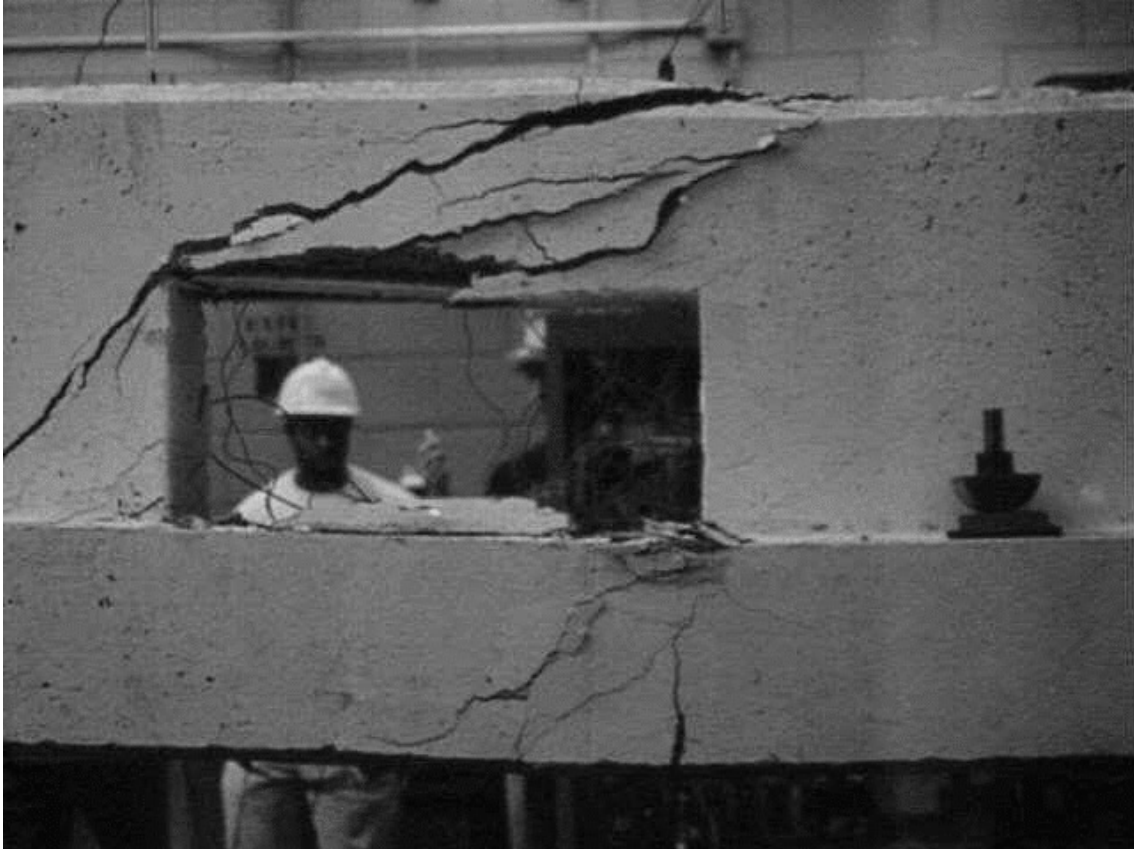
Figure 2.21 S2 at opening 1 after peak load (support to left in photograph)
