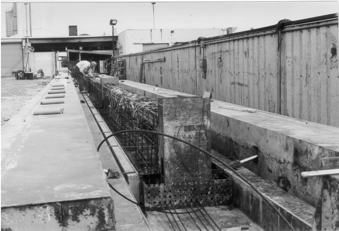
Figure 2.9 Fabricated cages in casting bed
