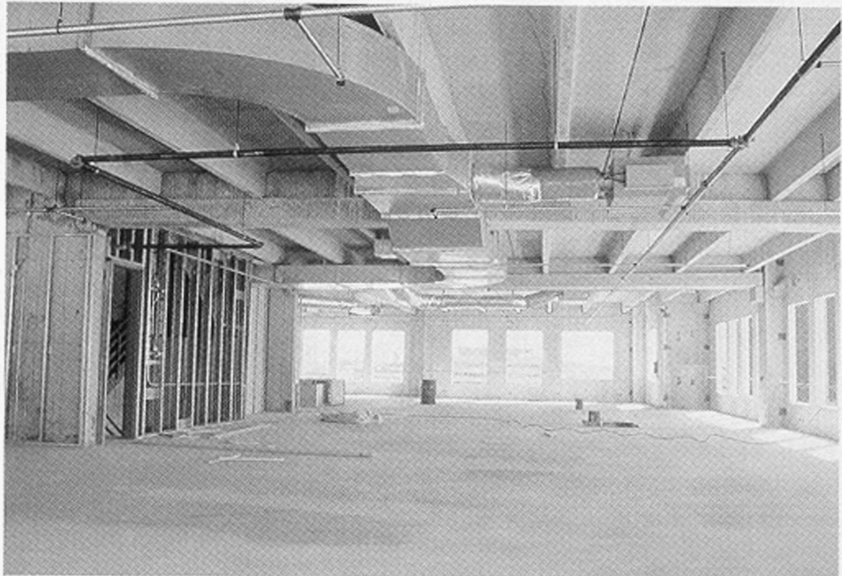
Figure 1.3 Office building constructed with the conventional system
