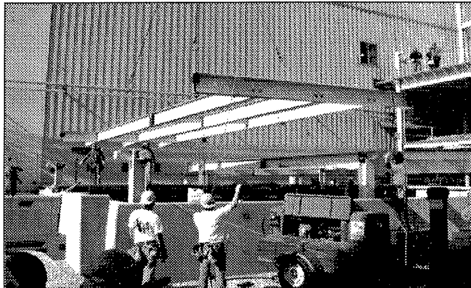
Figure 23. Bay During Erection.
