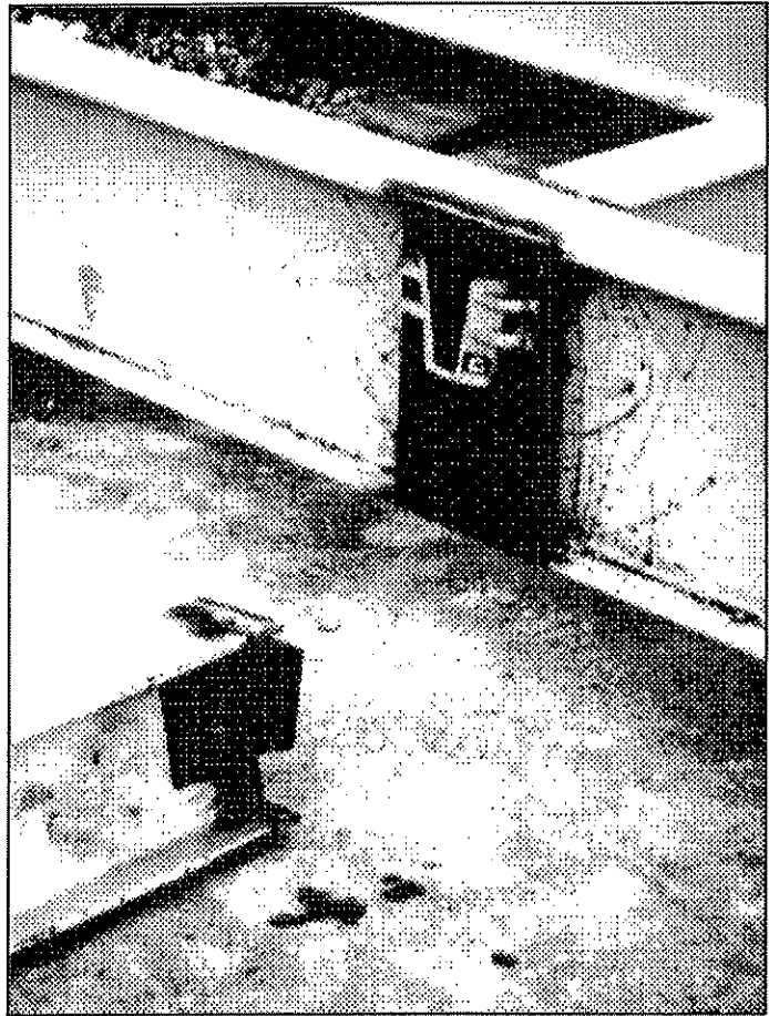
Figure 22. Members Prior to Erection.
