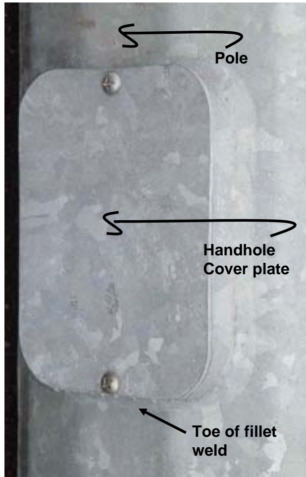
Figure 2.6 – Handhole detail
