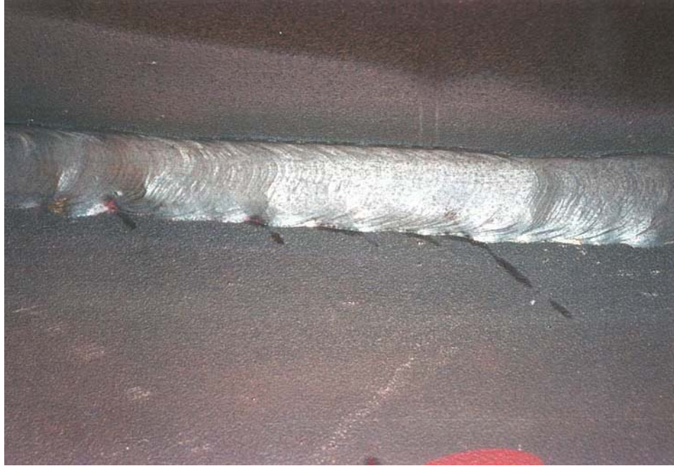
(a) Girder G2A
