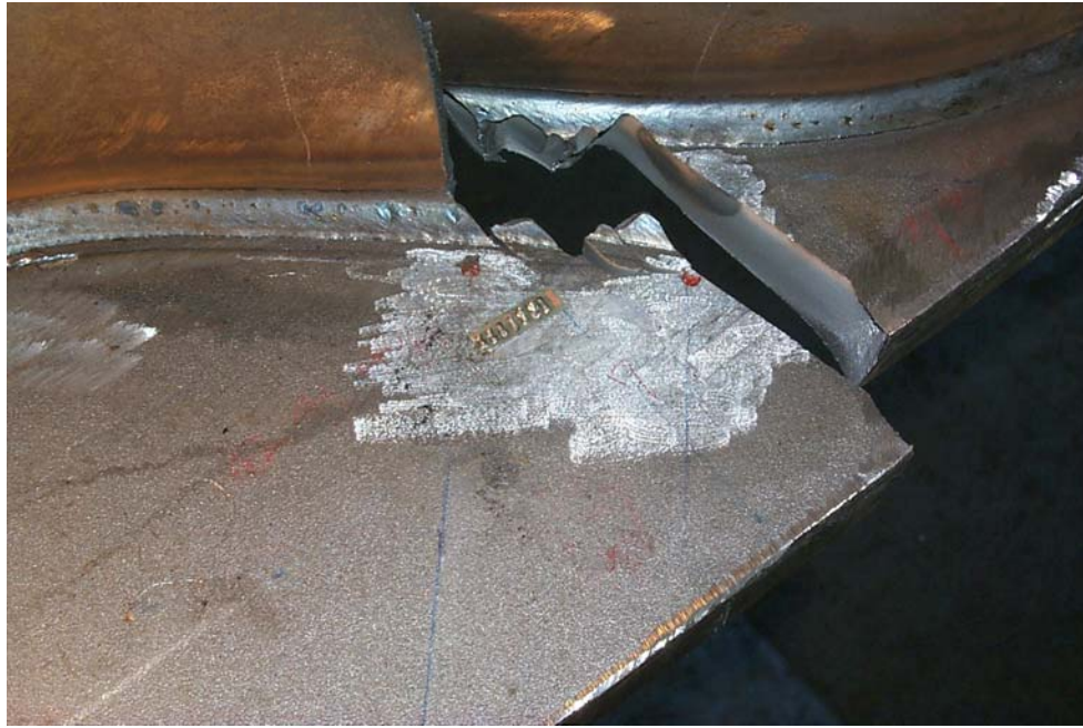
Figure 23. Failure of Girder G4B.
