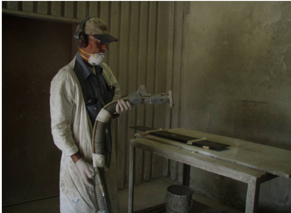
Figure 3.2 – Technician ready to apply DM
