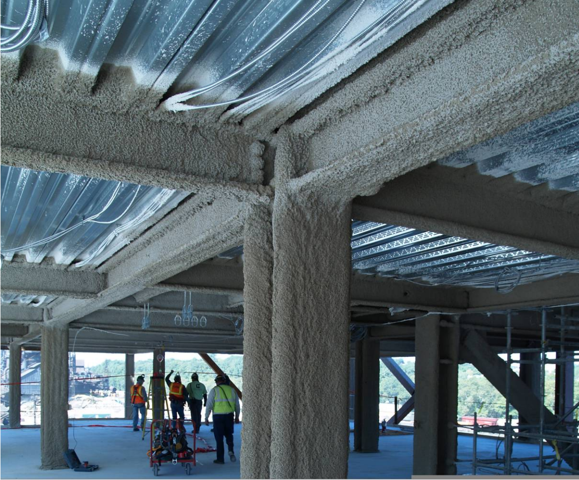
Figure 2.1 – Photograph of sprayed fire resistive material in building
