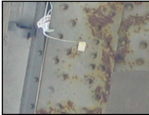
Figure 8 – Typical strain gage installed on bottom flange of a girder
