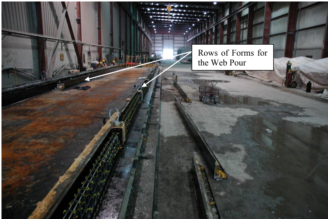
Figure 7-1: Prestressing Bed
