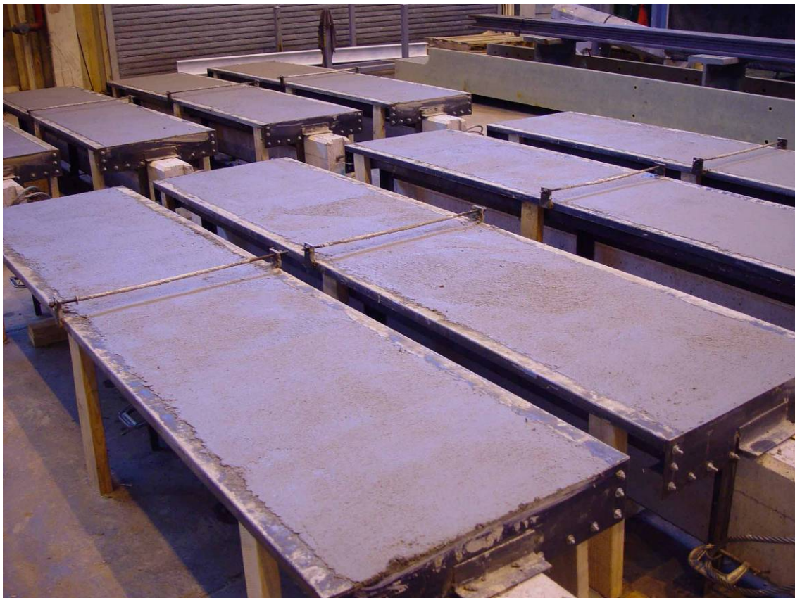
Figure 7-23: Beams After Slab Pour and Surface Finish
