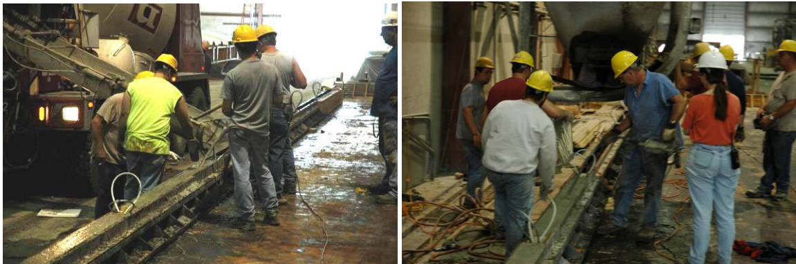
Figure 7-6: Placement of Web Concrete
