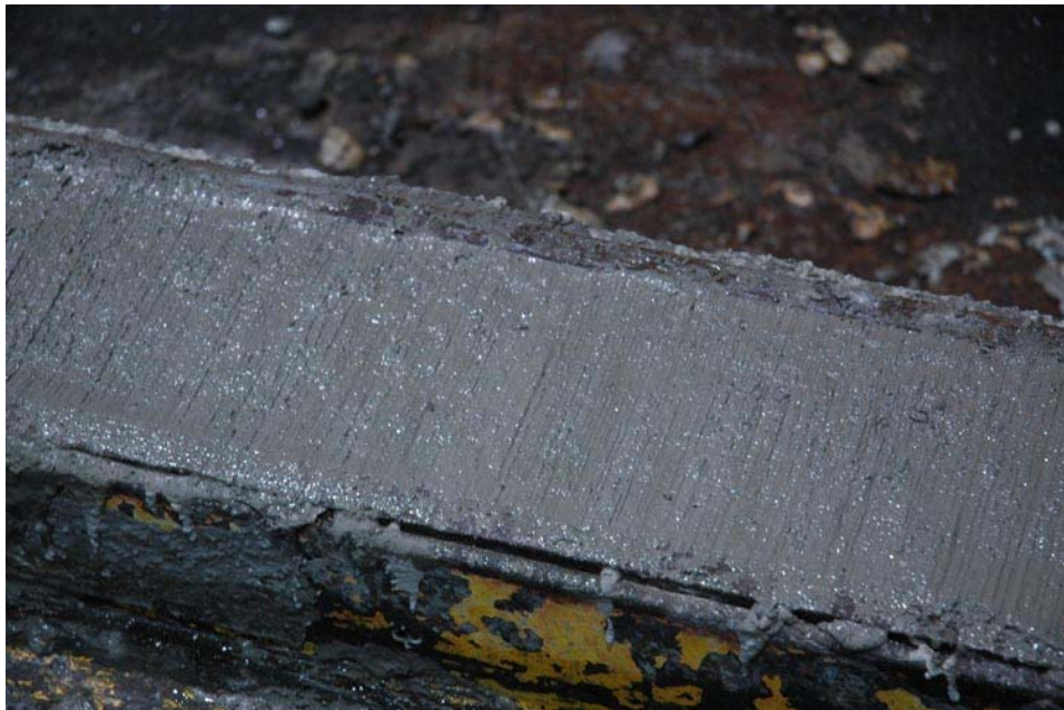
Figure 7-11: Broom Surface Finish
