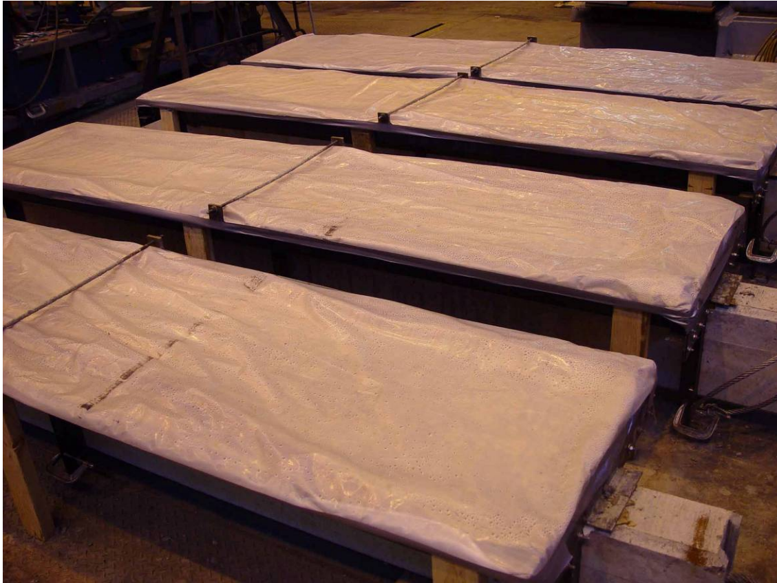
Figure 7-24: Slab Concrete Moist Curing
