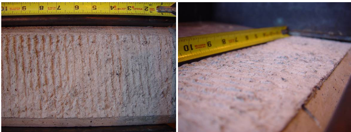
Figure 9-15: Rake Surface Finish – “Rough” [Specimen 6R7]
