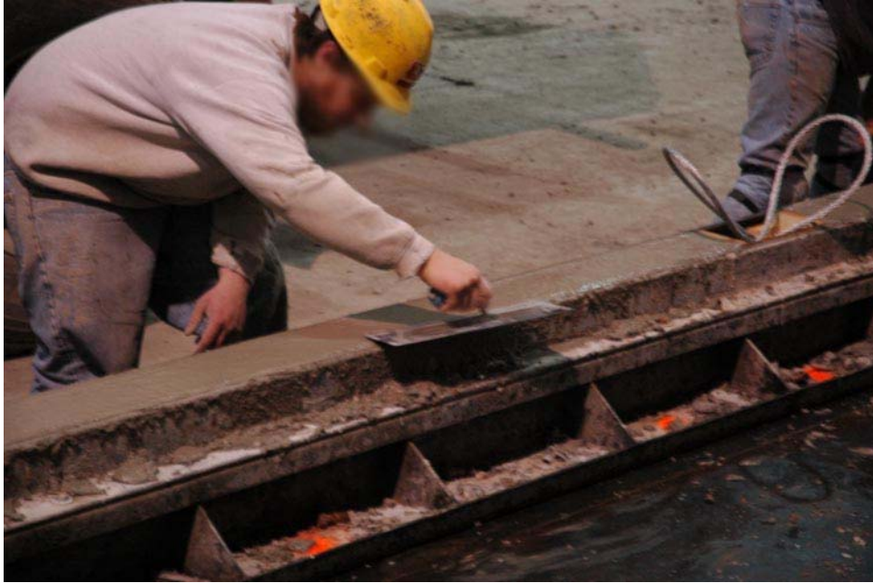
Figure 7-8: Applying a Smooth Surface Finish with a Hard Trowel
