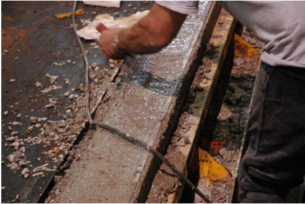
Figure 7-12: Applying the Rake Surface Finish
