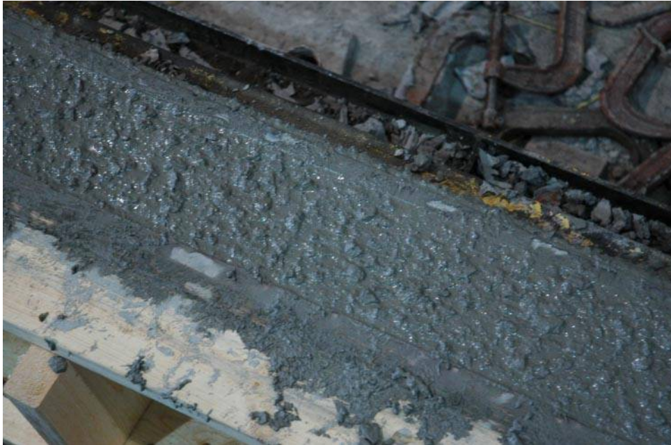
Figure 7-7: As-Placed Surface Finish
