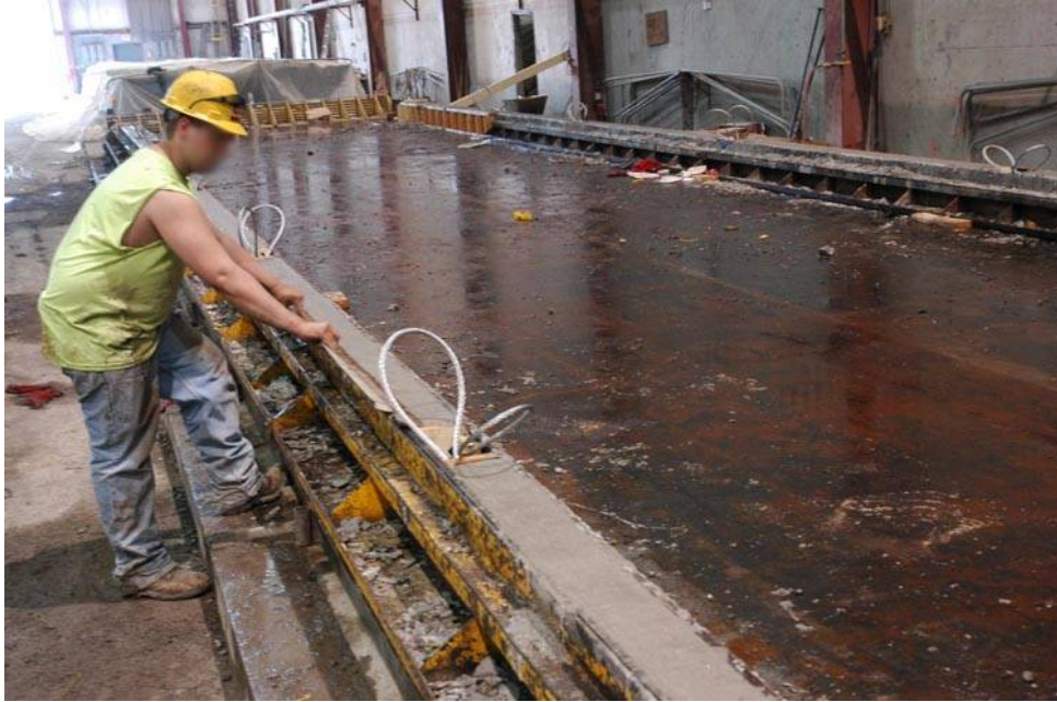
Figure 7-10: Applying the Broom Surface Finish
