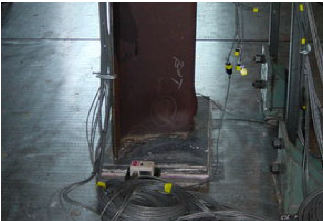
Figure 4-13 Local Buckling of Rib Wall near the Bottom of Column, Specimen SC
