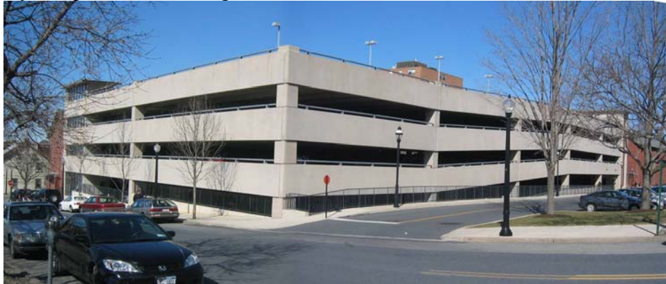
Figure 3-1: Lehigh University Campus Square Parking Garage (Southwest corner).
