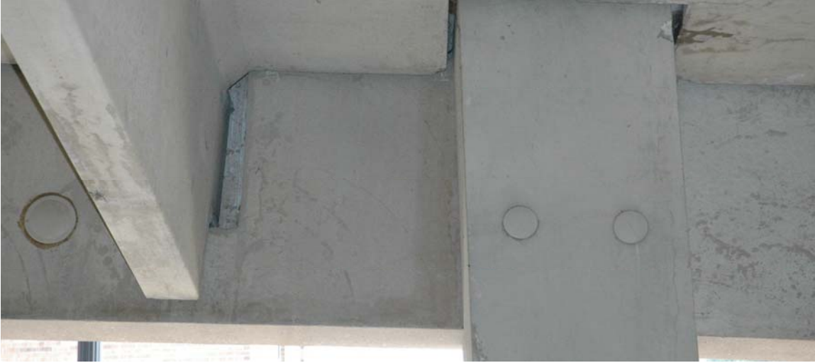
Figure 3-6: Exterior spandrel beam supporting double-tee.
