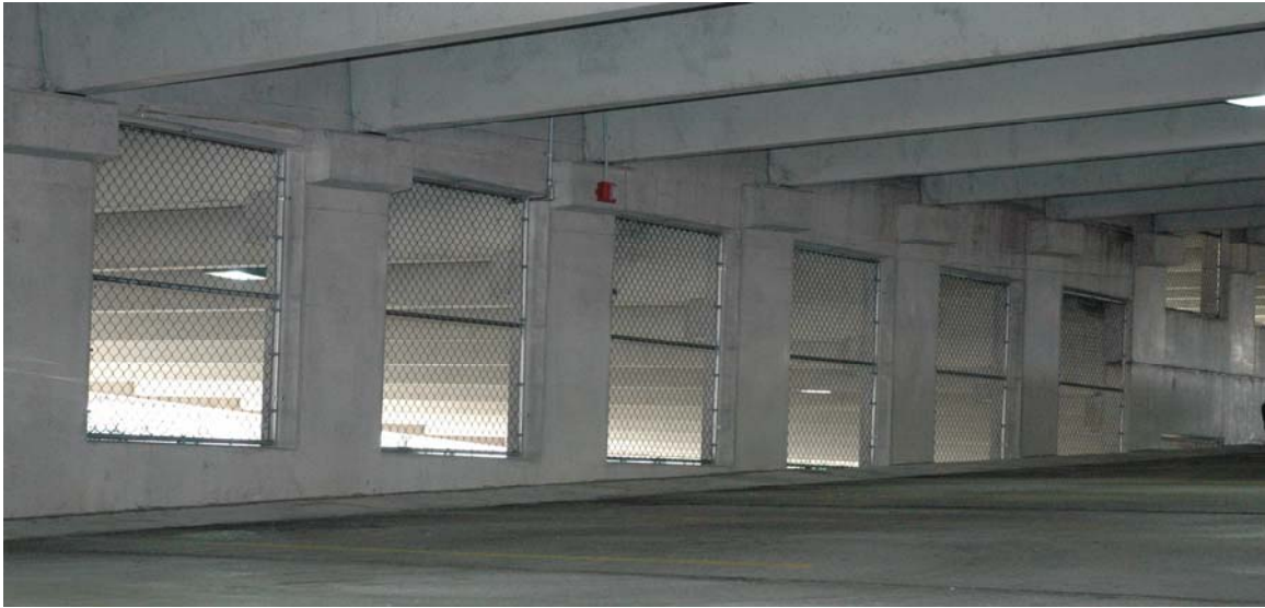
Figure 3-9: Photograph of the center wall of the prototype garage.
