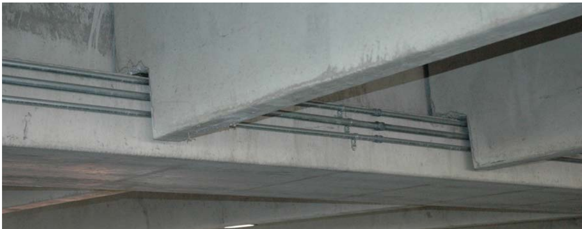
Figure 3-5: Inverted-tee spandrel supporting double-tee.
