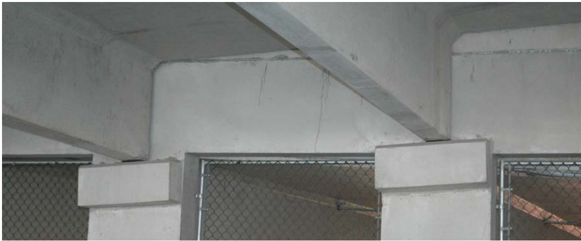
Figure 3-4: Corbels supporting double-tee.
