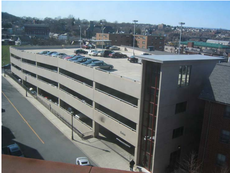
Figure 3-2: Lehigh University Campus Square Parking Garage (Southeast corner).
