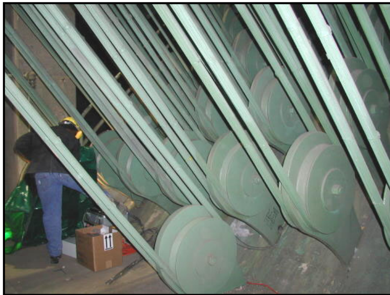
Figure 2 – Photograph of portion of eyebar assembly in southeast anchorage
