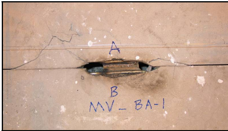
Figure 48: Specimen MV_BA-1 - condition of A-B connector at a shear load of 15.2 kips showing spalling of concrete
