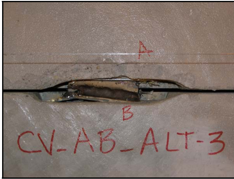
Figure 77: Specimen CV_AB_ATLUS-3 – deformation of “B” connector faceplate at a shear load of 14.0 kips (displacement of 0.6 inches)
