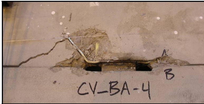
Figure 50: Specimen CV_BA-4 - spalling of top surface of panel at a load of 2.2 kips (displacement of 0.225 inches)
