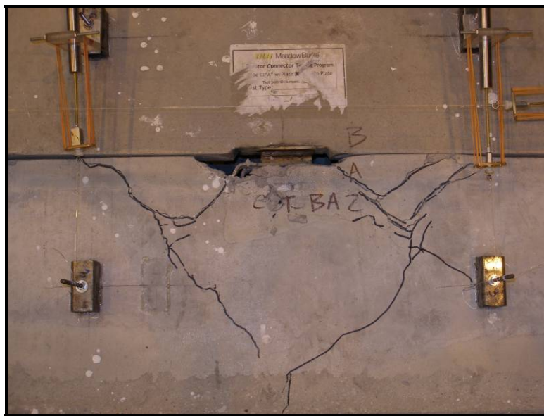
Figure 66: Specimen CVT_BA-2 – cracking and spalling of top surface at a shear load of 4.1 kips and a tension load of -1.0 kips (shear displacement of 0.3 inches)
