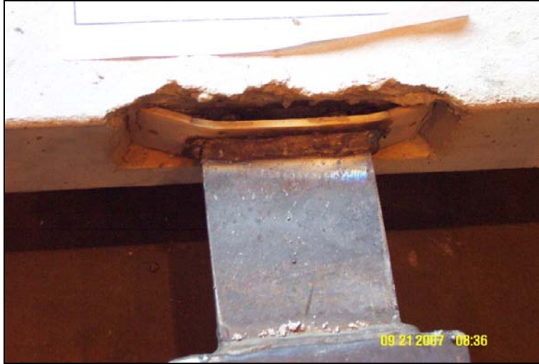
Figure 86: Bowing of connector plate
