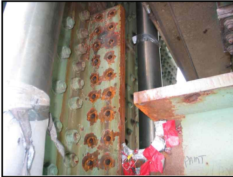
Figure 4.10 – Prototype retrofit at floorbeam FB77 with rivets removed
