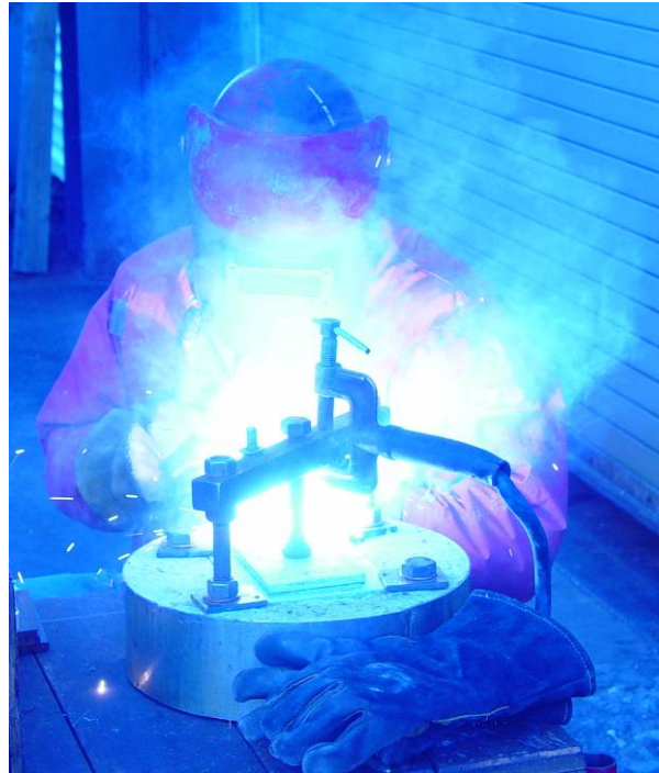
Figure 7.8: Outdoor Welding of Galvanized Steel
