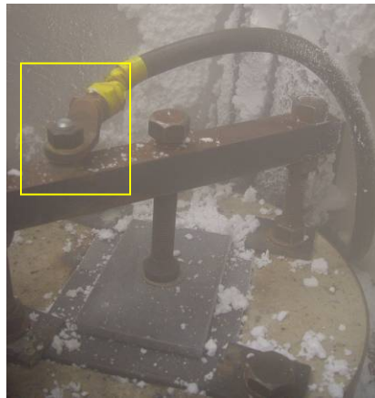
Figure 3.7: Welding Electrical Ground
