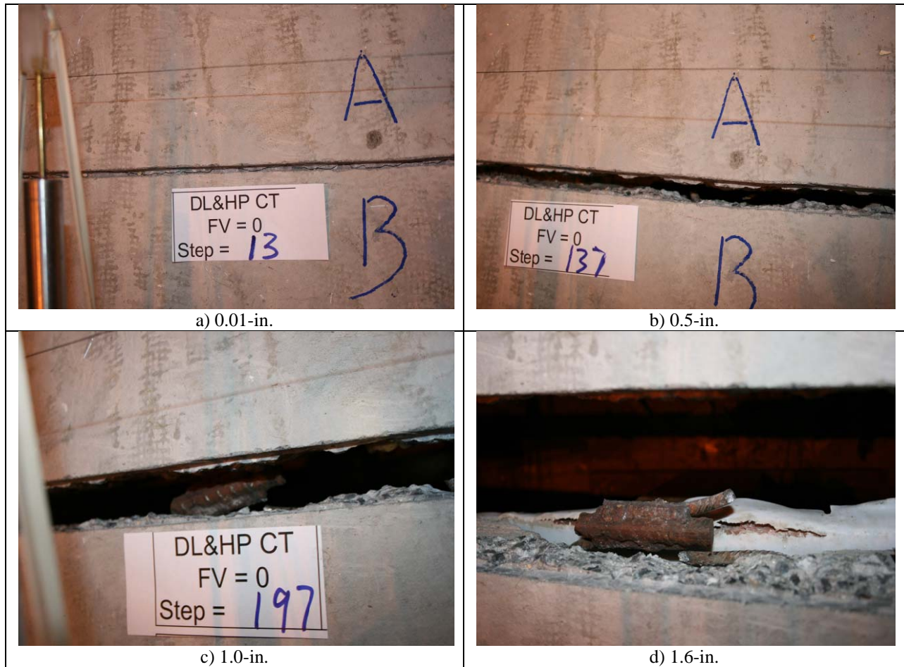
Figure 6-5: Damage state at various axial deformations.
