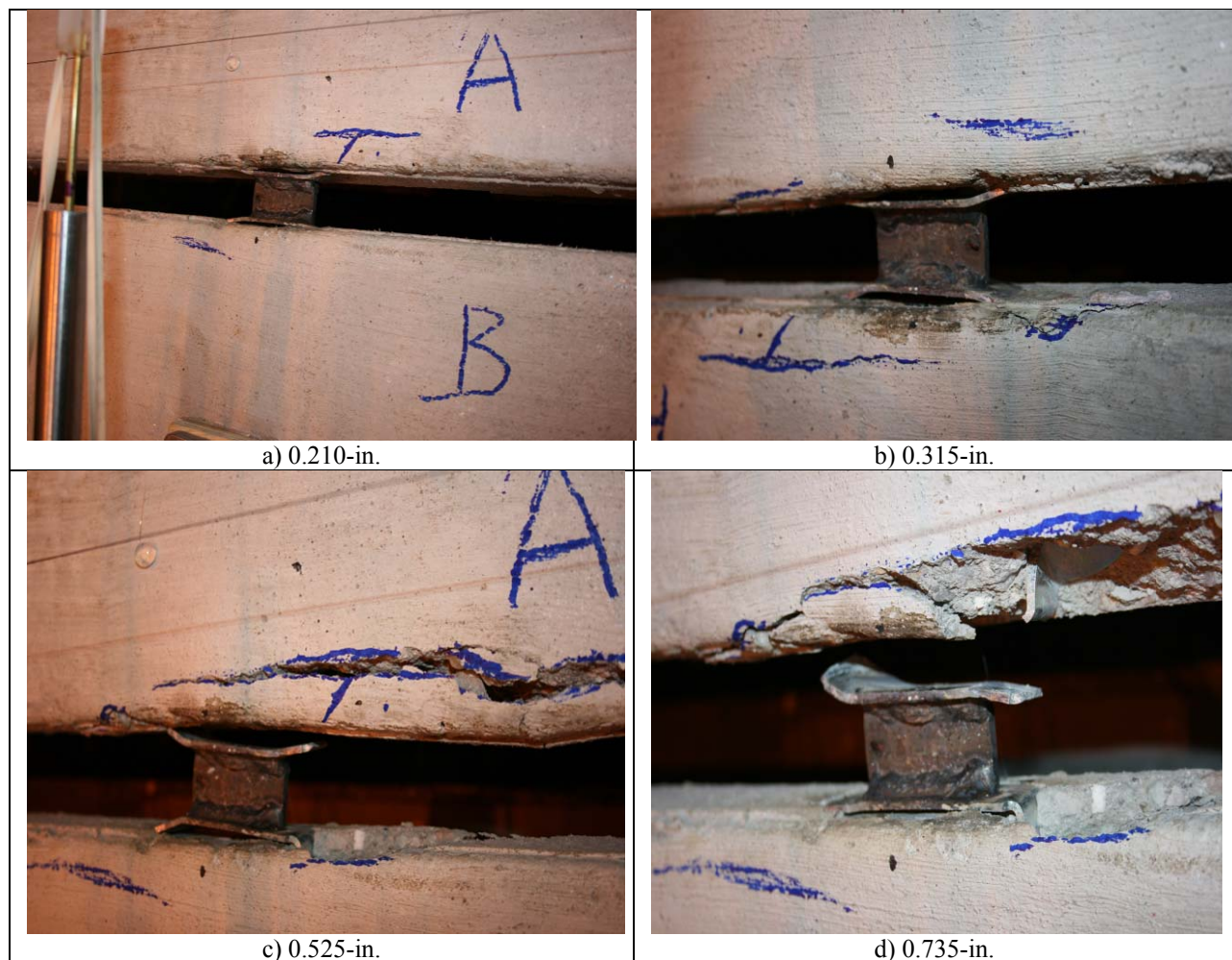
Figure 5-3: Damage state at various axial deformations.
