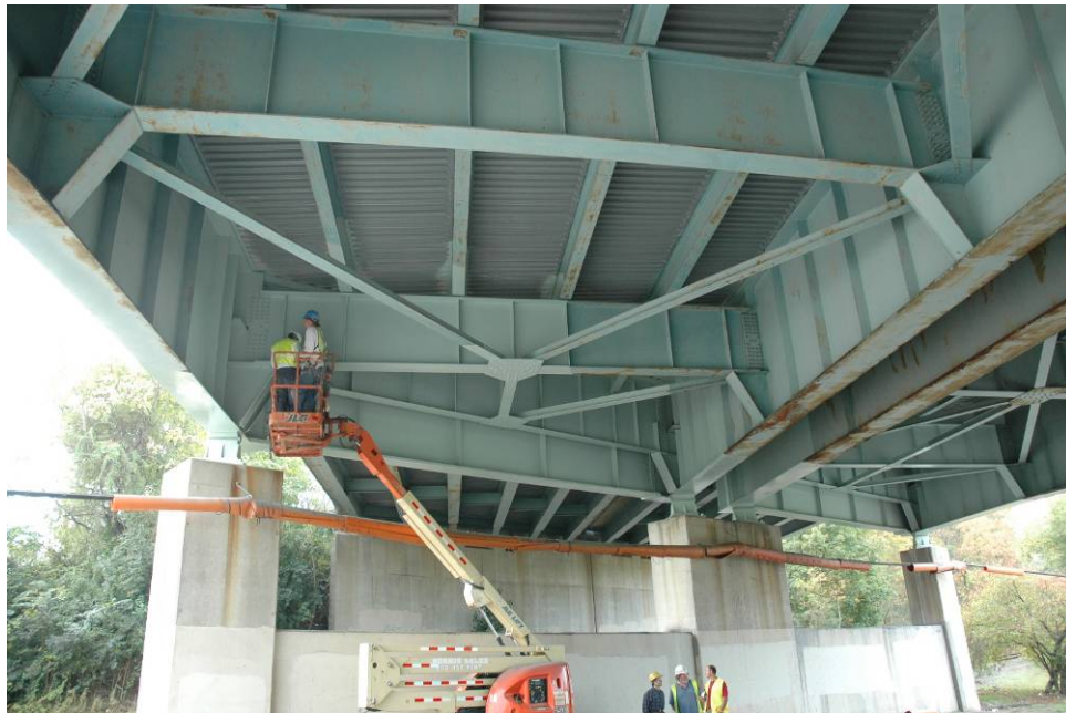
Figure 15 Access to underside of bridge deck
