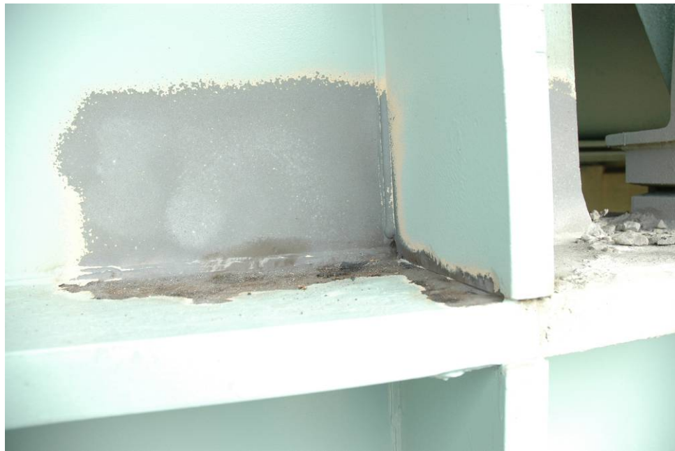
Figure 9 Bearing stiffener at bracket shelf plate
