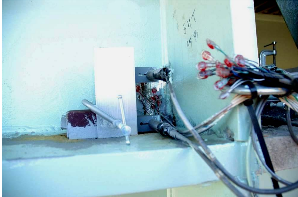
Figure 19 Arrangement of LVDTs on the span side of bearing stiffener
