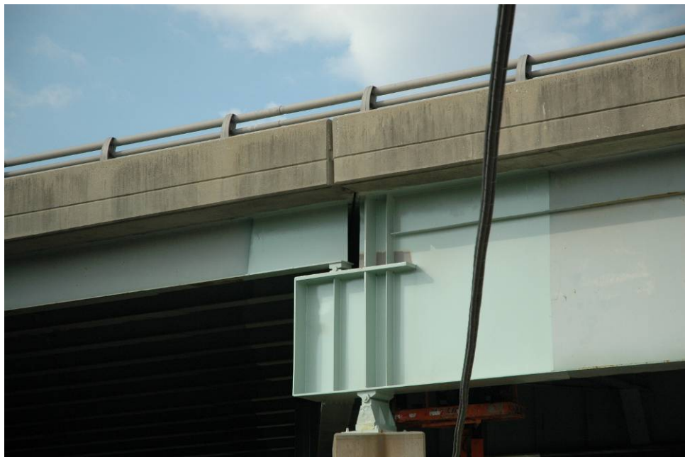
Figure 11 Seating of Span 1 on bracket projection from girder of Span 2
