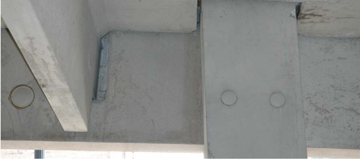
Figure 3-6: Exterior spandrel beam supporting double-tee (Bayreuther, 2006).
