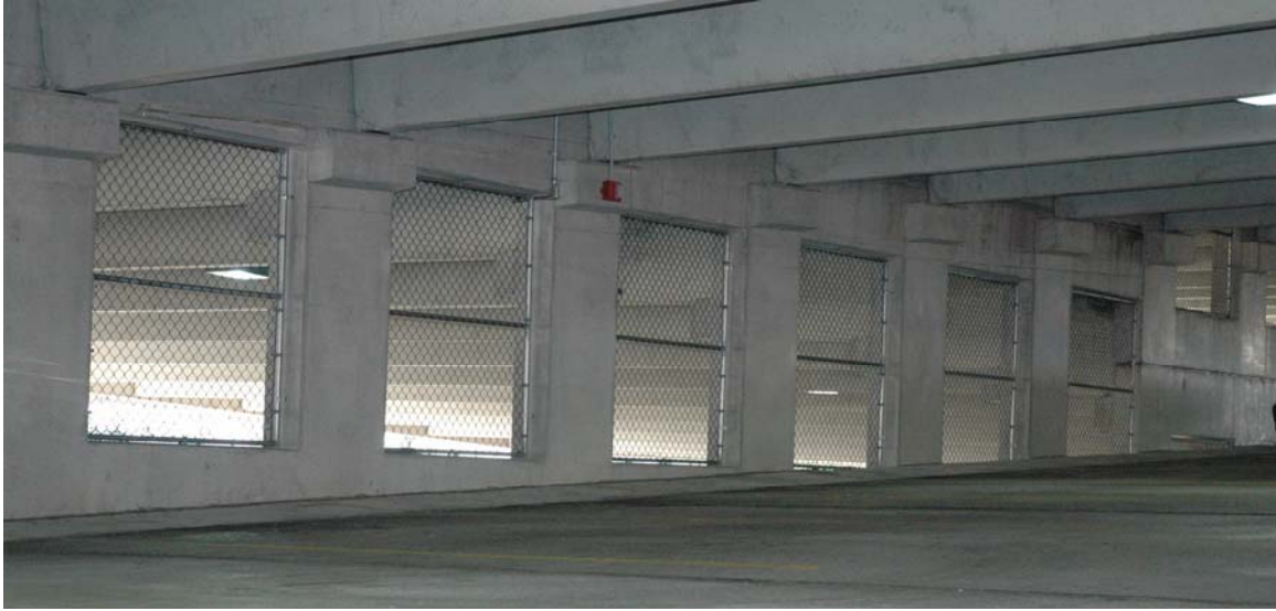
Figure 3-19: Image of the center wall of the prototype garage (Bayreuther, 2006).
