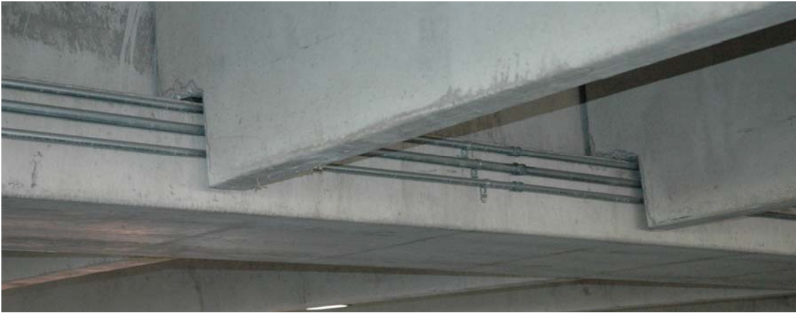
Figure 3-4: Inverted-tee spandrel supporting double-tee (Bayreuther, 2006).
