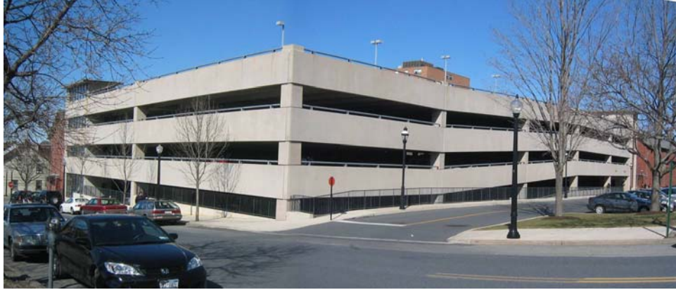
Figure 3-1: Lehigh University Campus Square parking garage (southwest corner) (Bayreuther, 2006).
