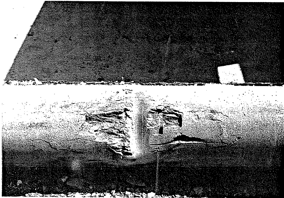
Figure 3.80. Closeup View of Exposed Grout Beneath Dent (a) Before, and (b) After Removing Loose Grout, Specimen A3.
