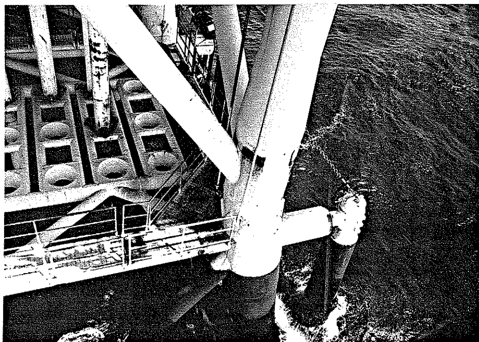
Figure 1.1 (a) and (b). View of diagonal bracing members framing into platform jacket leg at waterline.
