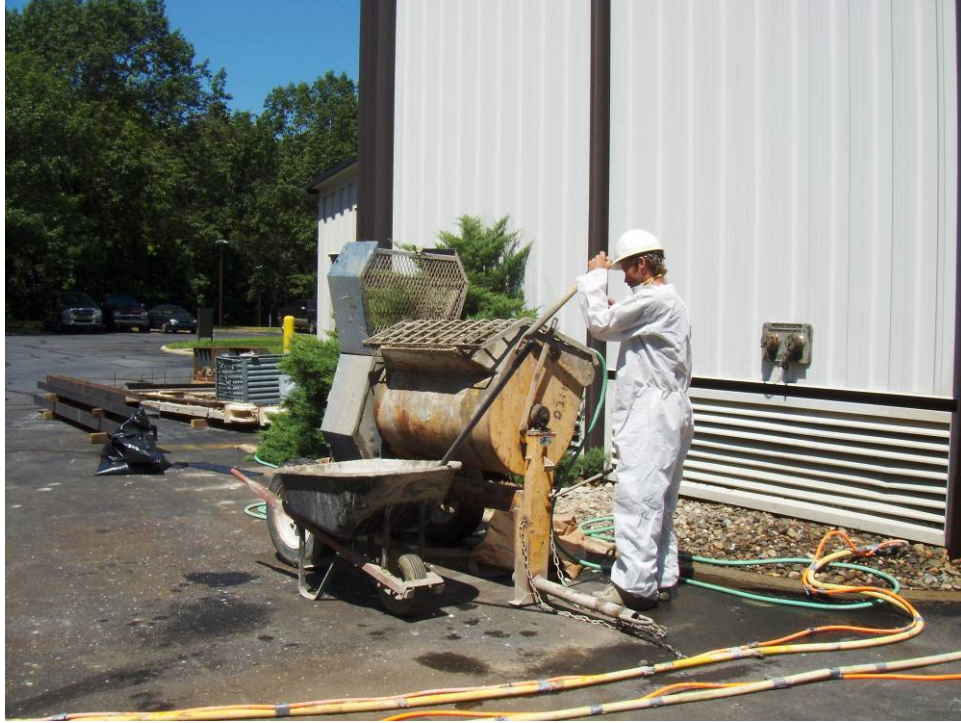
Figure 3.13 – Mixing WM with water
