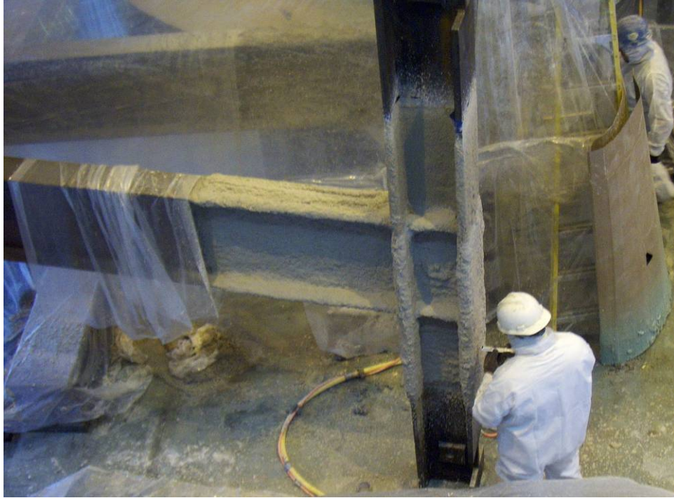
Figure 3.18 – Technician checking the thickness of the WM
