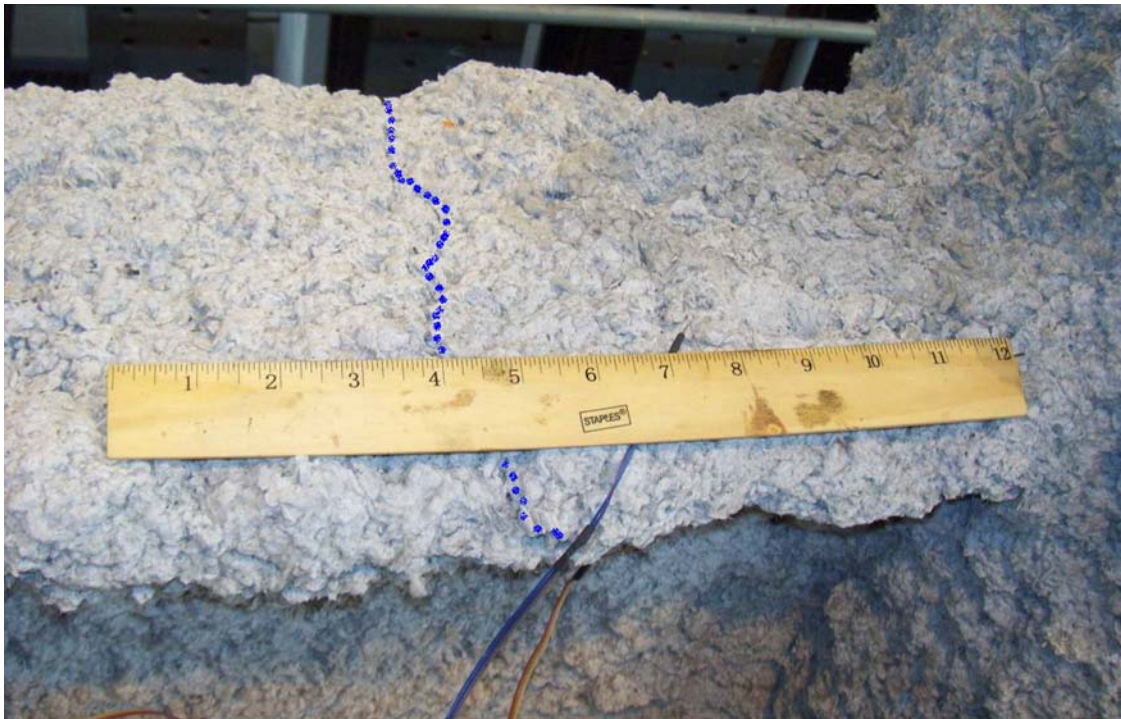
Figure 4.49 – Transverse crack in top flange of DM assemblage during post-testing inspection
