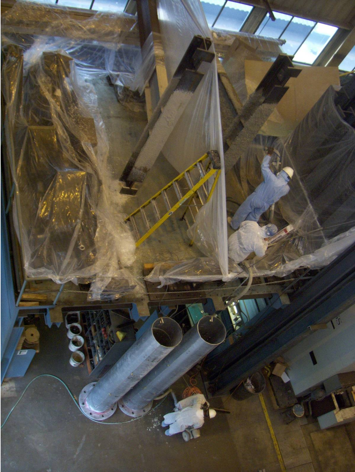
Figure 3.12 – Staging area for application
