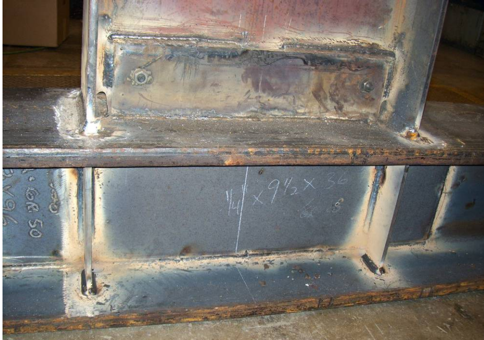
Figure 3.7 – Photograph of connection region after steel fabrication
