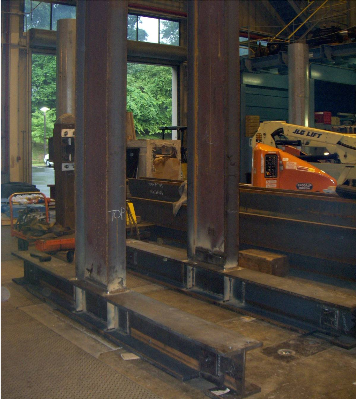
Figure 3.6 – Specimens after steel fabrication and before sprayed fire resistive material application
