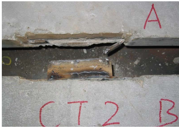
Figure 25: Damage at end of test
