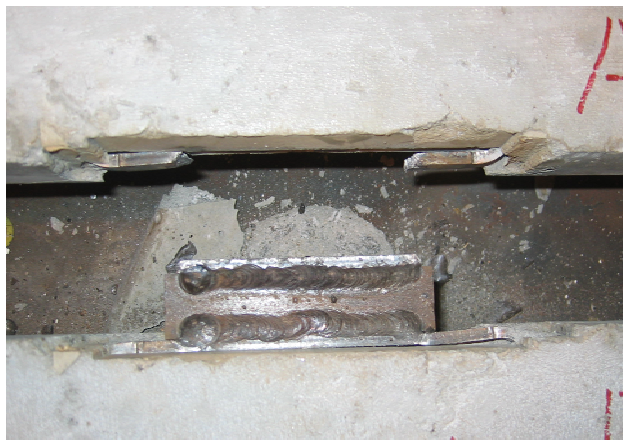
Figure 22: Damage at end of test
