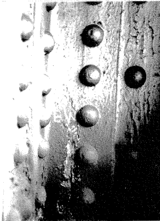
Figure 4. Fatigue Cracked Connection Angle
