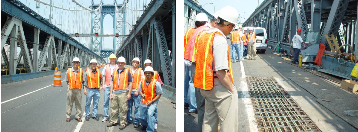
Figure 2: PITA REU students visit Manhattan Bridge renovation project
