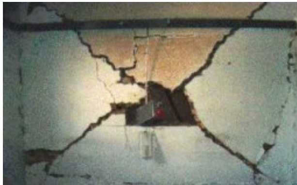
Figure 5: Wall Impact Test at RMCS
