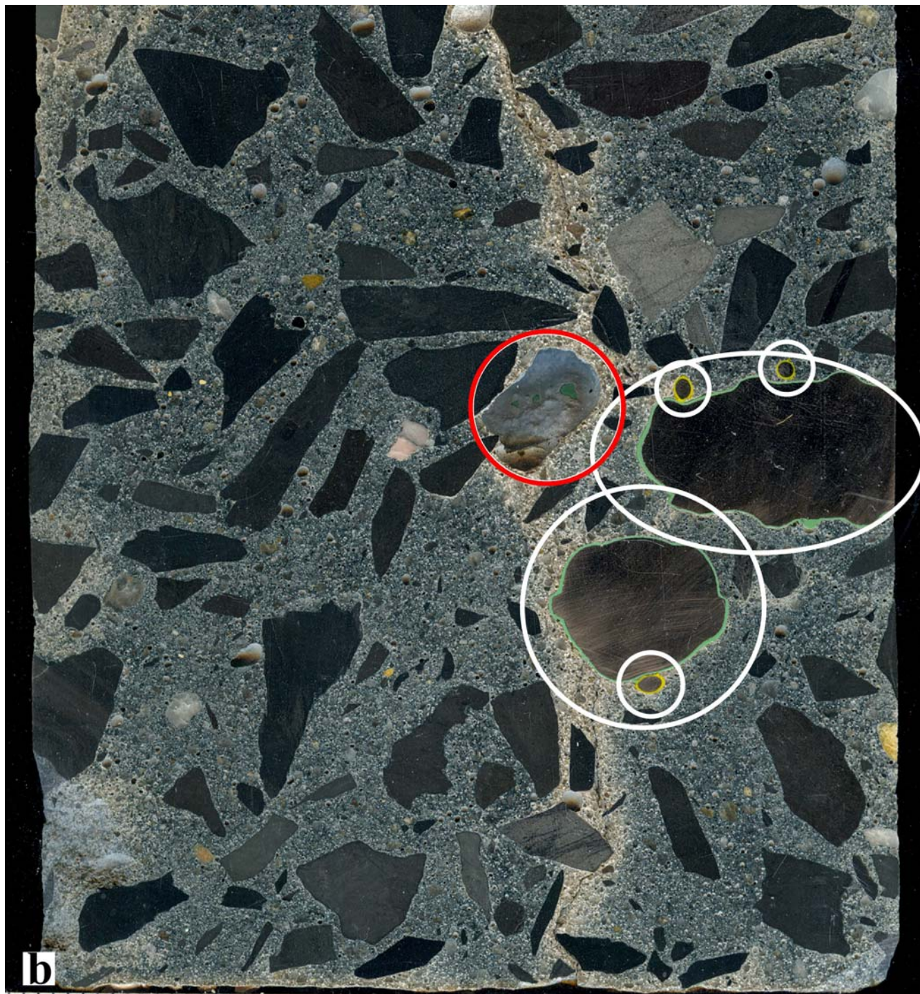
Figure 5B (Core 2) – Boxed Area "b" in Figure 5. No. 5 bars (large circle and ellipse) are green epoxy-coated, and tie-wires (small circles) are yellow epoxy-coated. Within the red circle is a large entrapped air void. The vertical crack circumscribes most aggregate particles and extends to the core bottom.
