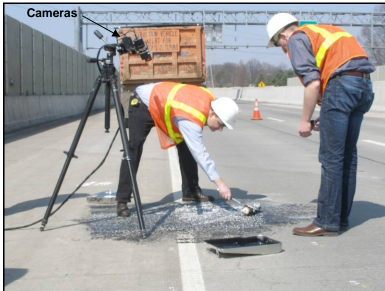
Figure 2.10 – Application of random speckle pattern to concrete deck surface
