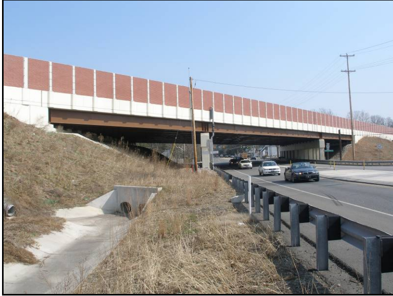
Figure 1.2 – View of SR309 bridge over Church Road looking east
