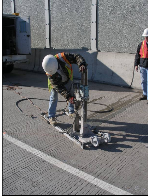
Figure 3.1 – Coring operation during removal of Core #1
