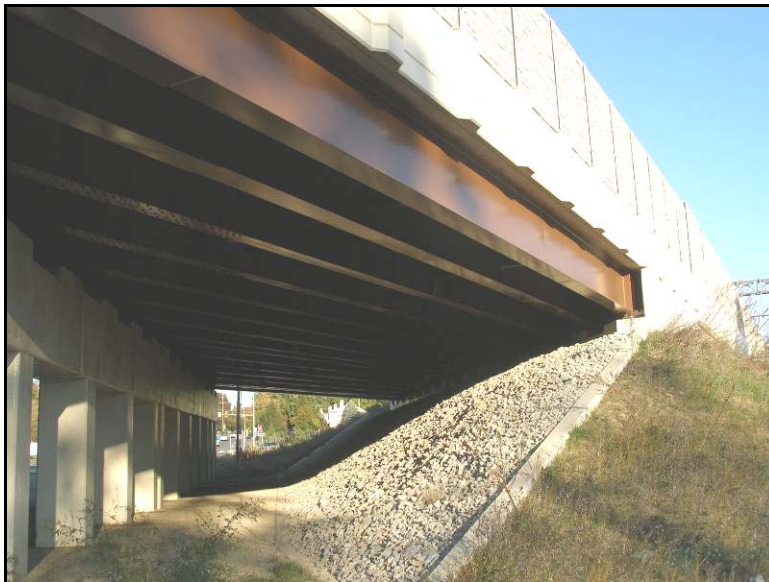
Figure 1.3 – View of SR309 bridge over Church Road looking northwest at Abutment 2
