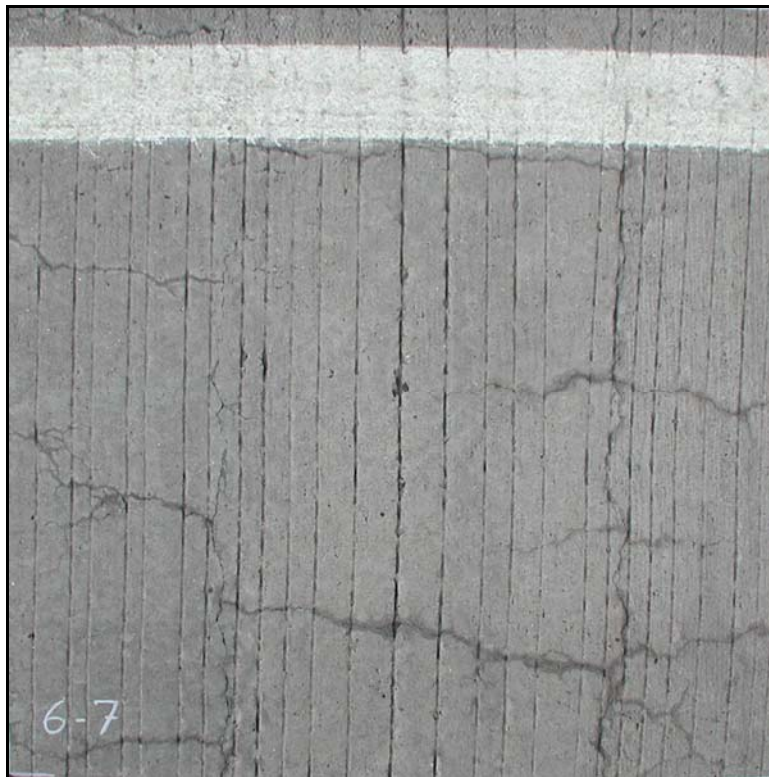
Figure 2.4 – Image of Square 6-7 in negative moment region after correction for perspective using Photoshop
