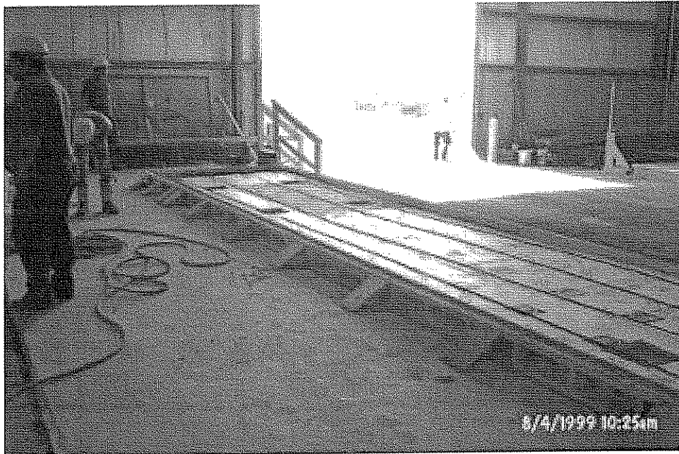
Figure 3.10 Placement of the back wythe prestressing strands.
