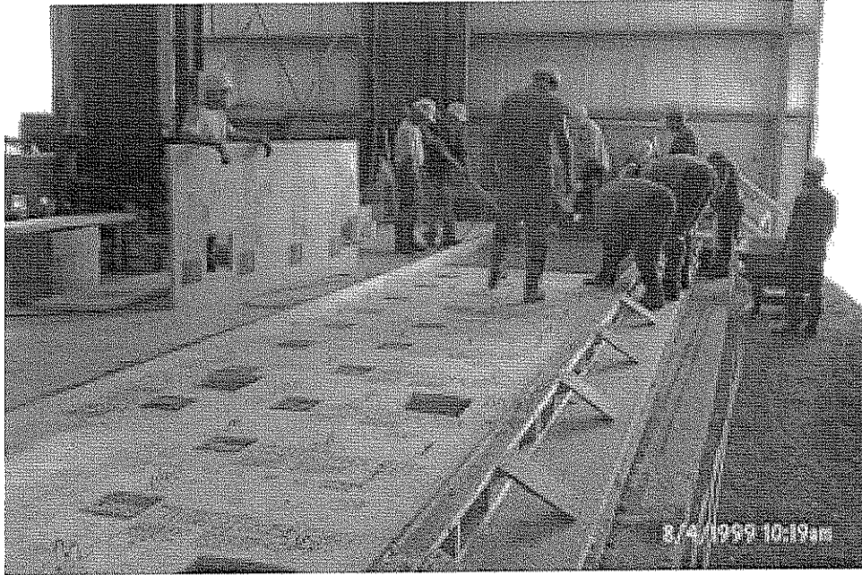
Figure 3.9 Placement of the steel M-tie connectors.
