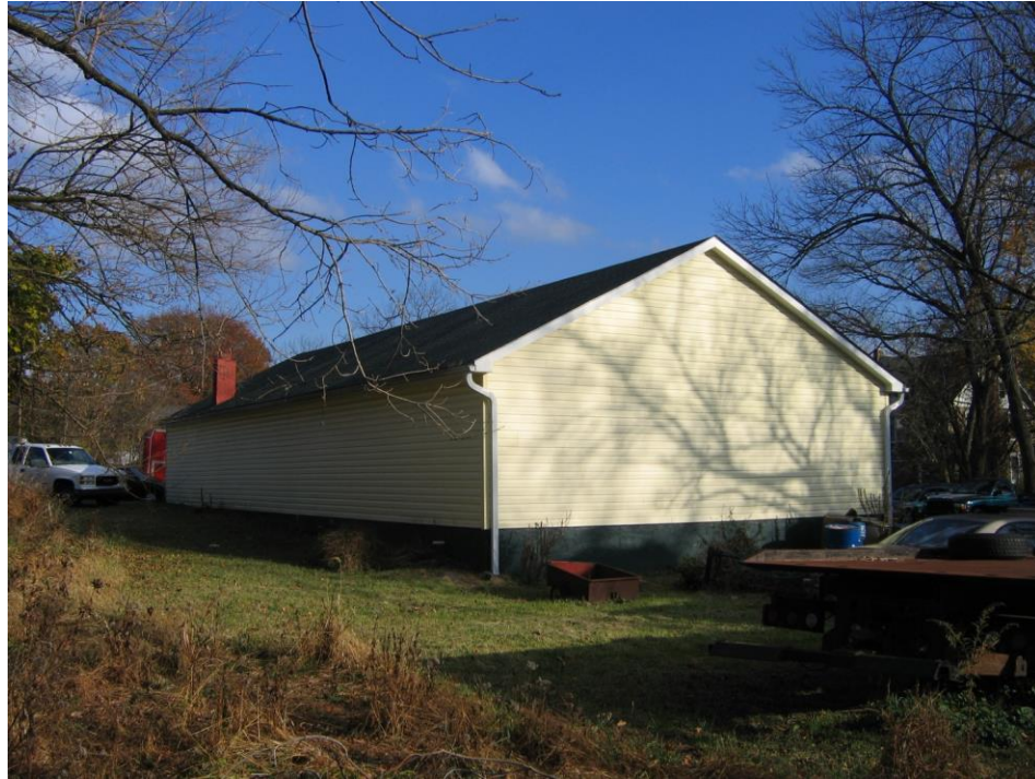
Figure 4.1 - H. S. Mill Canning Company - Former Site. This is the original site of the H. S. Mill Canning Company in Springtown, Pennsylvania. The present automotive repair facility sits upon the original foundation of the former cannery. Photograph taken by the author in April 2014.
