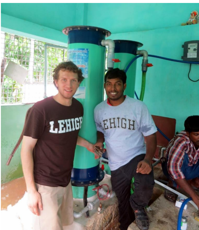
Figure 5.7. Anil Shaw and Mike German installing an SAC-Fe system in Binimaypara (N. 24 Parganas, West Bengal); a technician from Ramkrishna Water Mission is partially off-screen.
