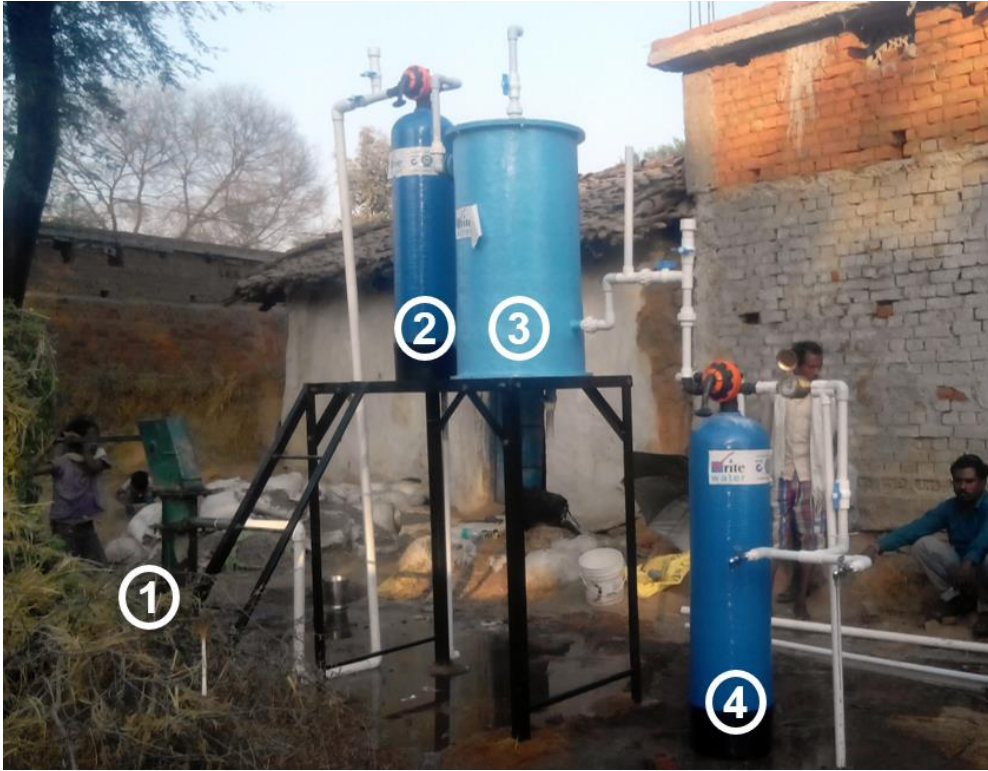
Figure 7.3. Original HAIX-NanoZr installation by Rite Water in Nuapada, Odisha. Note from Left-Right: 1) Handpump; 2) Column 1 (WAC resin); 3) storage tank/passive decarbonator; 4) HAIX-NanoZr.
