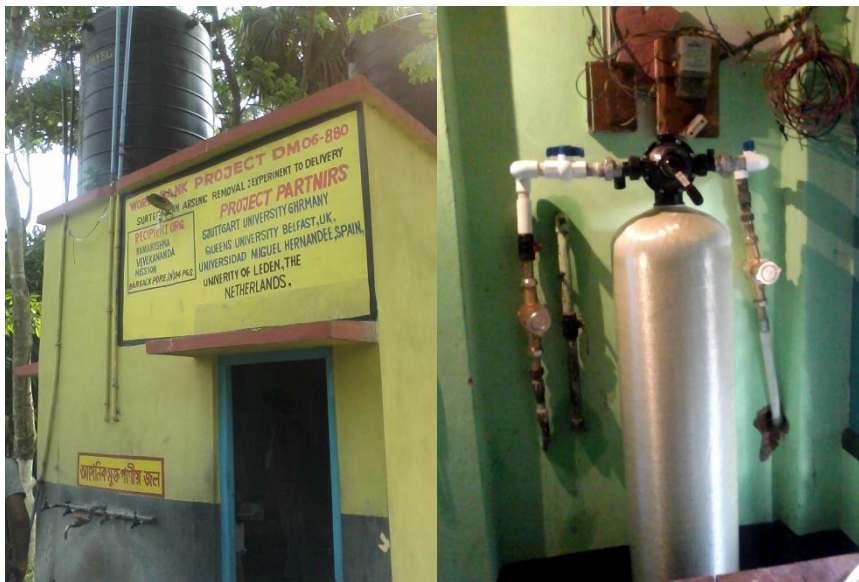
Figure 3.16. A) Building containing the original SAR system (L) and B) the post-treatment HAIX-NanoZr column placed in series after SAR treatment (R).
