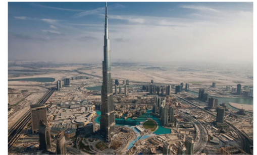
Figure 8: As the tallest building in the world, Burj Khalifa towers above all other buildings in Dubai, creating a dramatic skyline.
