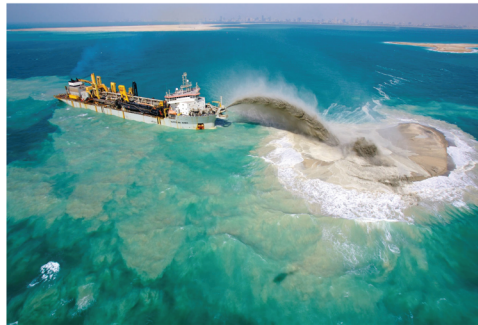
Figure 7: Dredging ship spraying sand to construct The Palm Islands.
