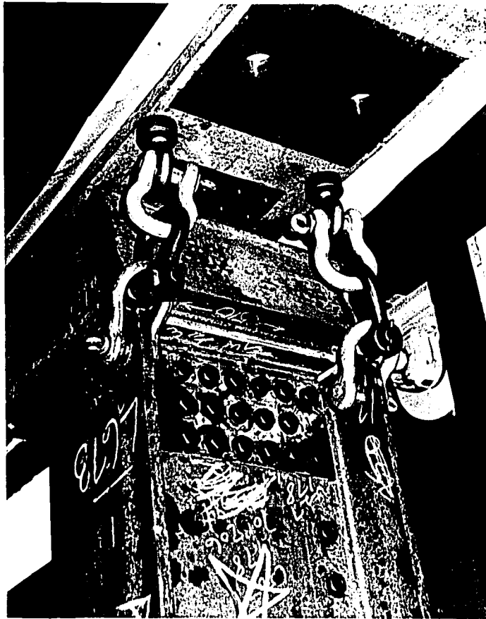
Fig. 13 Panel Lifting Arrangement
