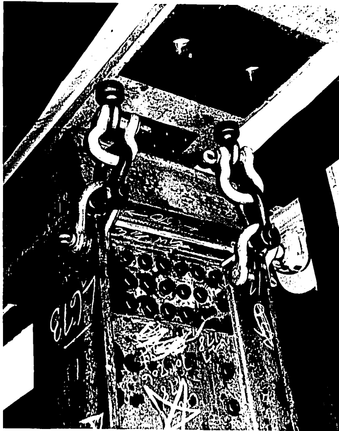
Fig. 13 Panel Lifting Arrangement
