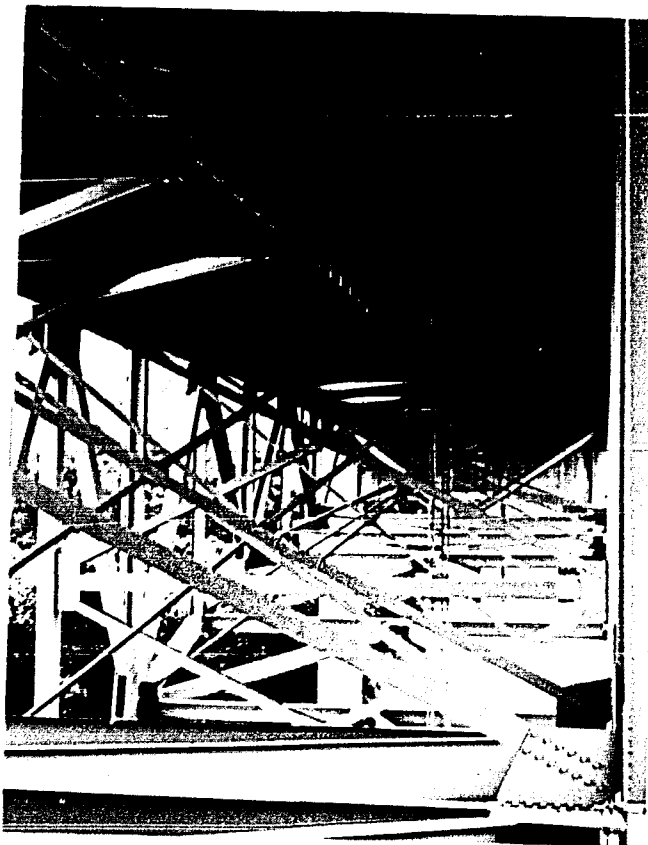
Figure 6 - View of the Kittanning Bridge under-deck truss spans.
