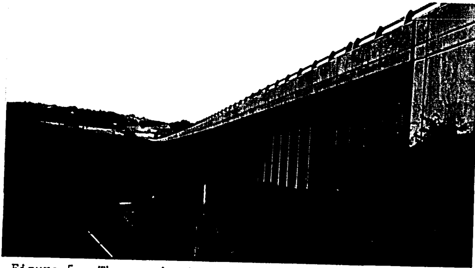
Figure 5 - The north girder span of the Kittanning Bridge viewed from the west.
