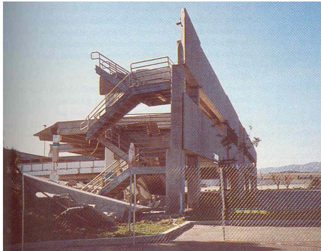
Figure 2.17. Collapsed parking garage (Iverson and Hawkins 1994)
