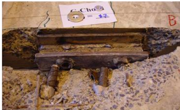
Figure 4.36. Damage state at 1.98-in shear opening
