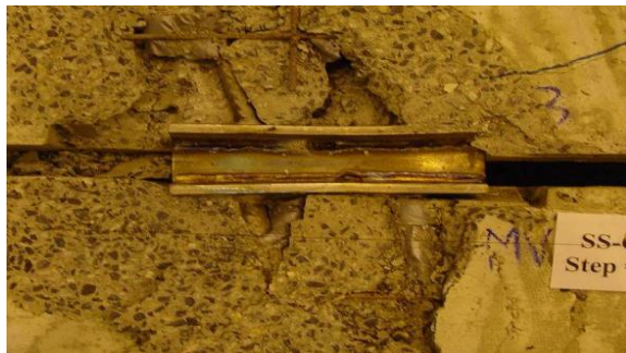
Figure 4.39. Damage state at 4.5-in shear opening
