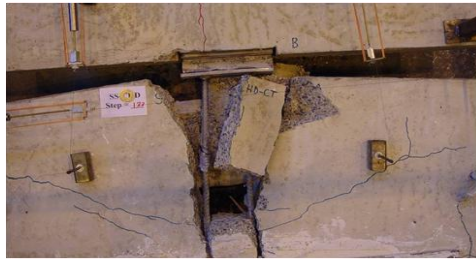
Figure 4.19. Damage state at 2.0-in tensile opening
