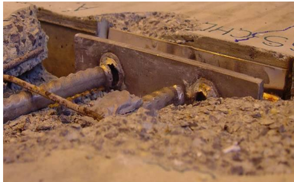
Figure 4.40. Damage state at 2.15-in shear opening
