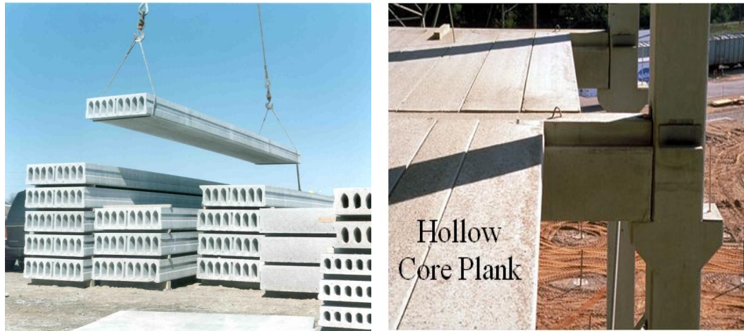
Figure 2.1. Precast hollow core planks
