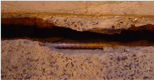
Figure 4.13. Damage state at 2.0-in tensile opening
