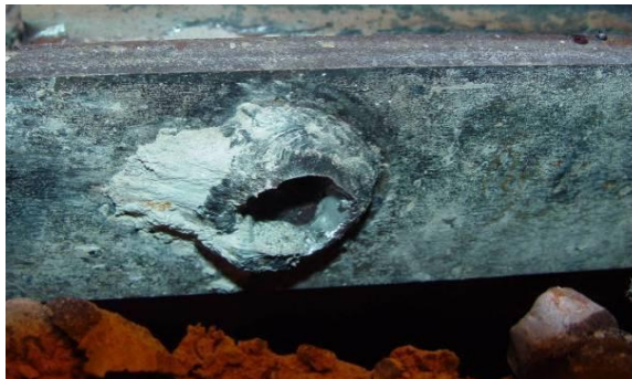
Figure 4.34. Damage state at 3.5-in shear opening
