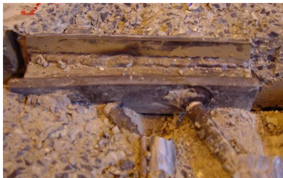
Figure 4.35. Damage state at 3.5-in shear opening
