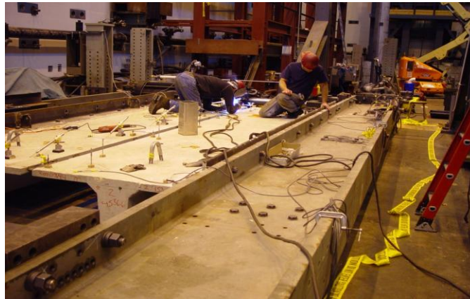
Figure 7.2. Field welding of connections between panels
