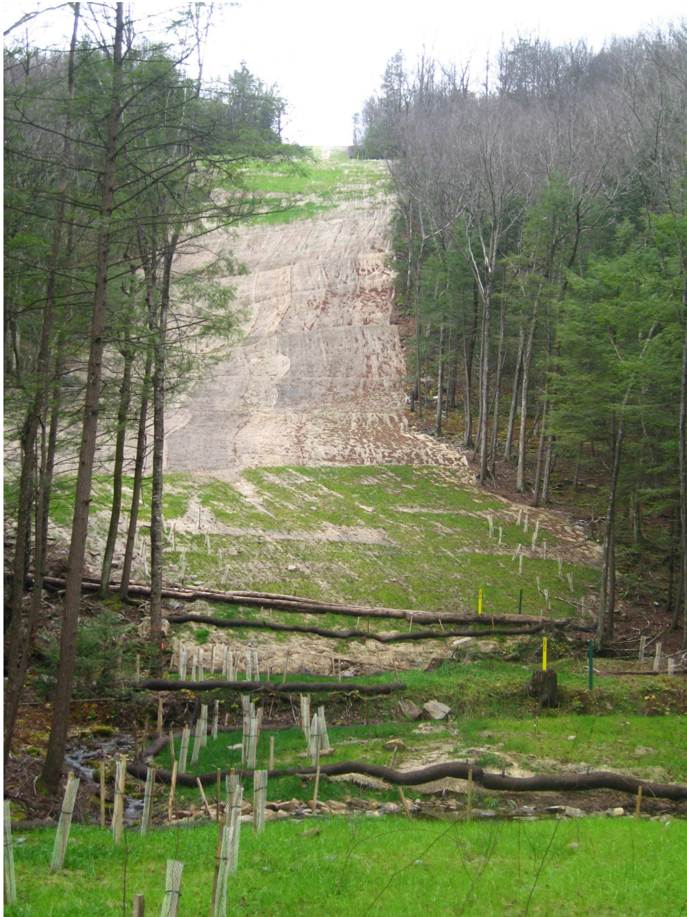
Figure 3.1 - Forest Clearing: The forest was removed for the installation of a new natural gas pipeline. There is the possibility of stream sedimentation due to run off and the possibility of temperature rise due to clearing.
