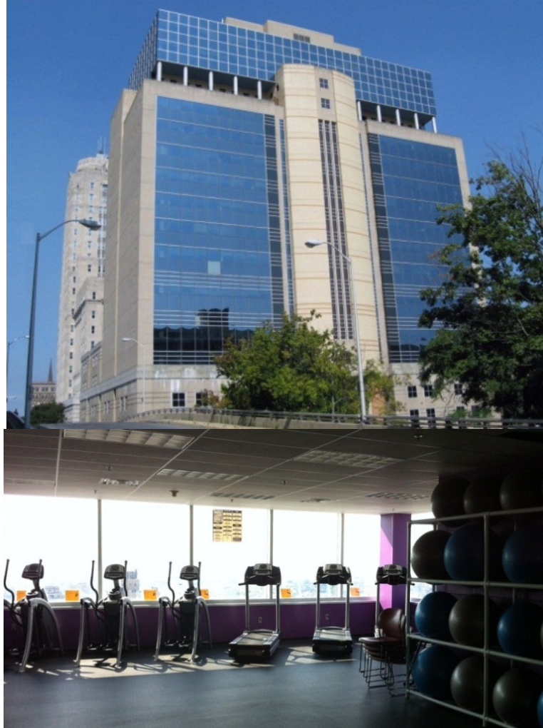
Figure 6.3. Test bed structure and 16 th floor exercise room
