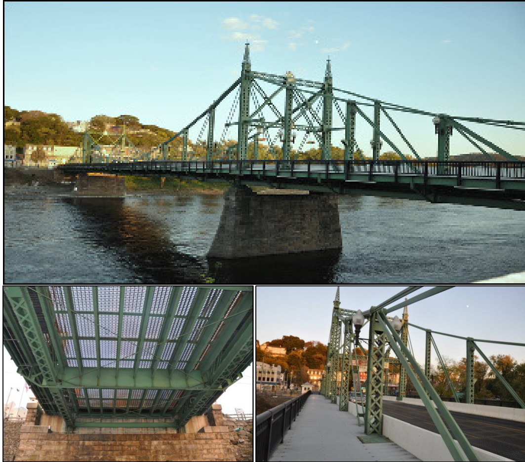
Figure 7.1. A view of the Northampton St. Bridge
