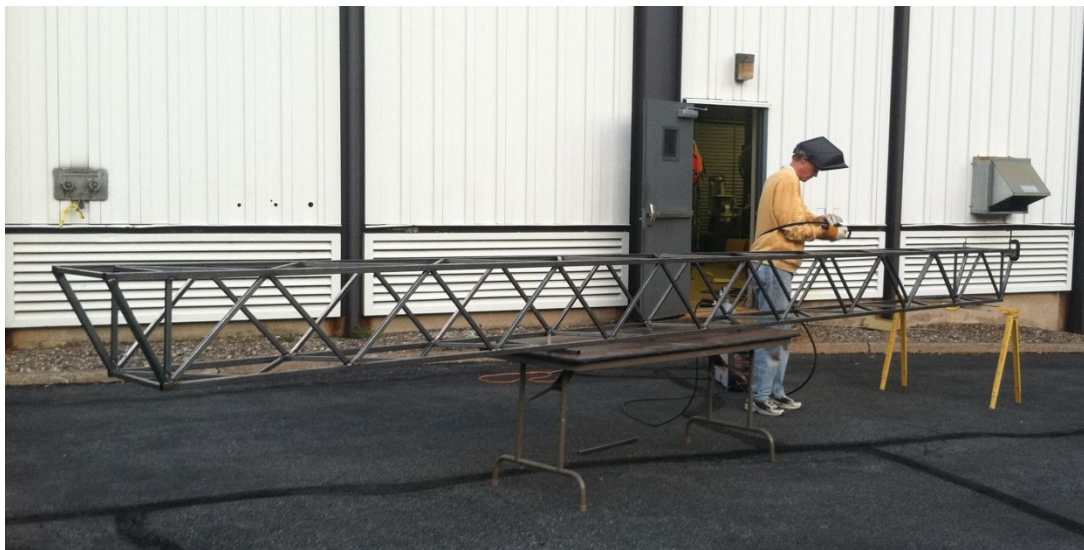
Figure 36: Finish Welding Support Truss
