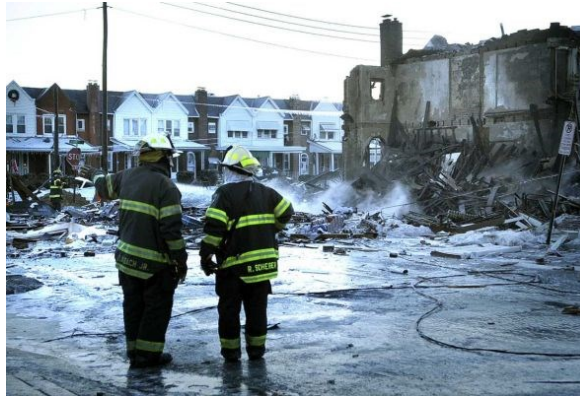
Figure 33 The demolished houses in Allentown's accident [6].
