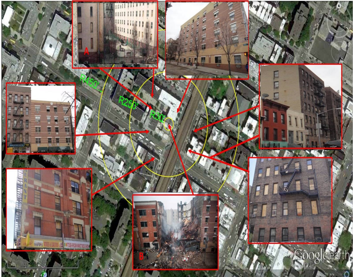
Figure 41 Associated damage between 30 to 250 ft [9]
