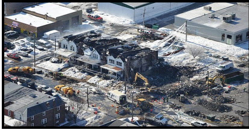
Figure 17 Allentown's natural gas explosion [3].
