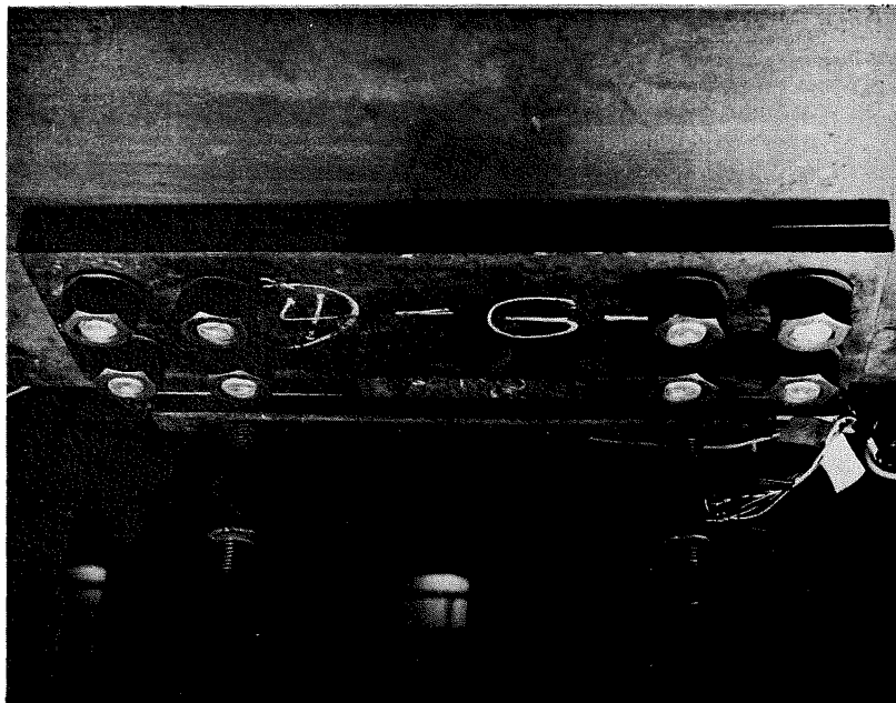
Fig. 42 High-Strength Bolted Splice across a Through Crack Originating at a Type VII ca Detail (Viewed from Beneath Girder 3)
