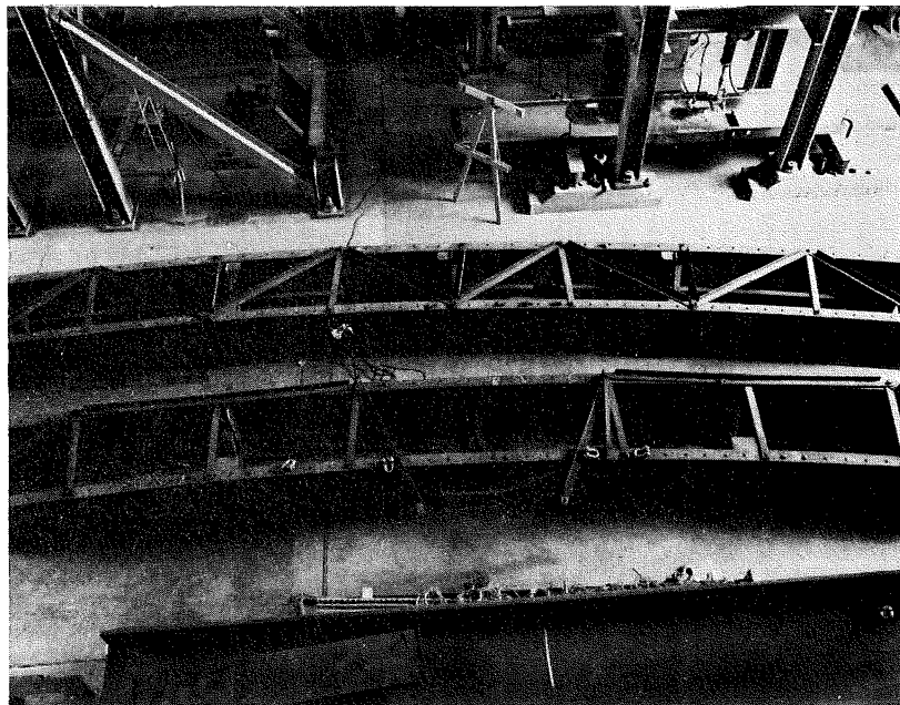
Fig. 8 Girders 1 and 2 during Preparation for Testing Showing Temporary Top Lateral Bracing System
