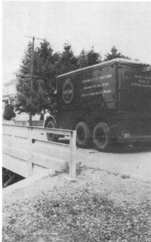
Fig. 9 Scale Truck. Total Weight 37,600 lbs.
