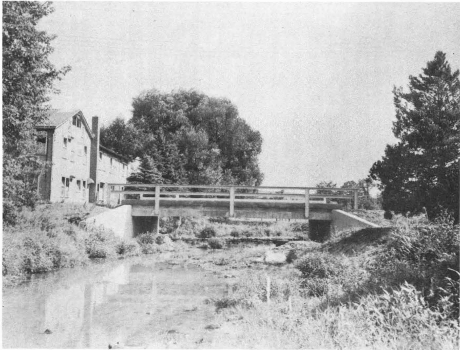
Fig. 2 Side View of the Bridge
