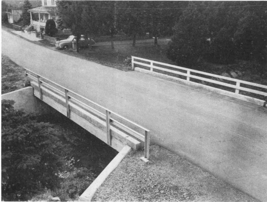
Fig. 1 General View of the Test Bridge
