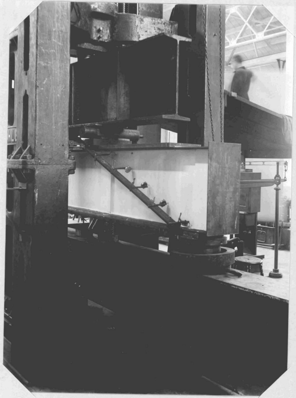
Fig. 29 - Loading Arrangement for Beam WB-4, A Reinforced Bethlehem B28-91 Section
