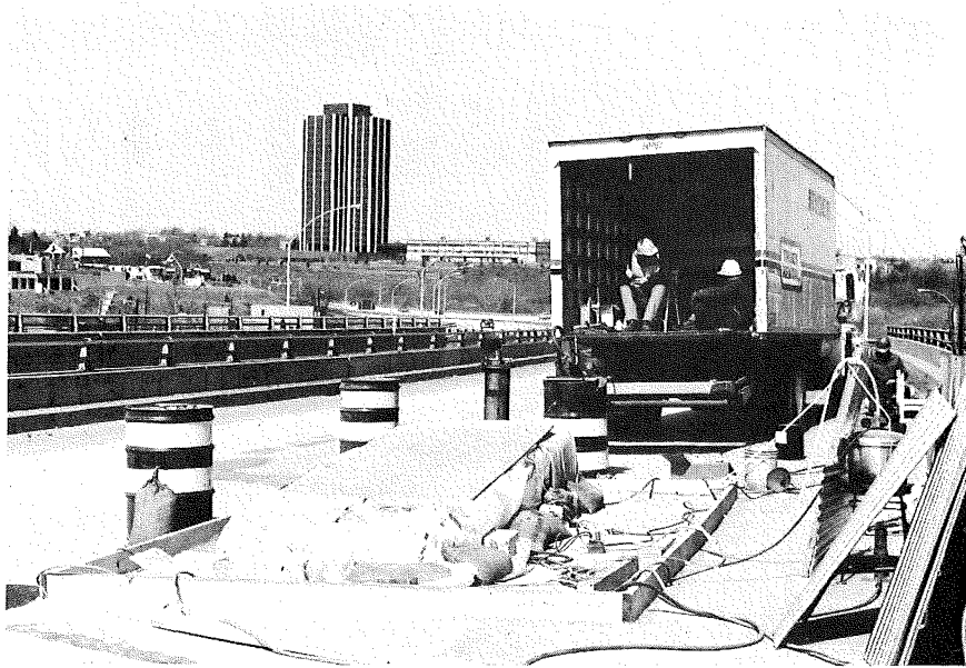
Fig. H-30 Polymerization Step. Note Insulation.
