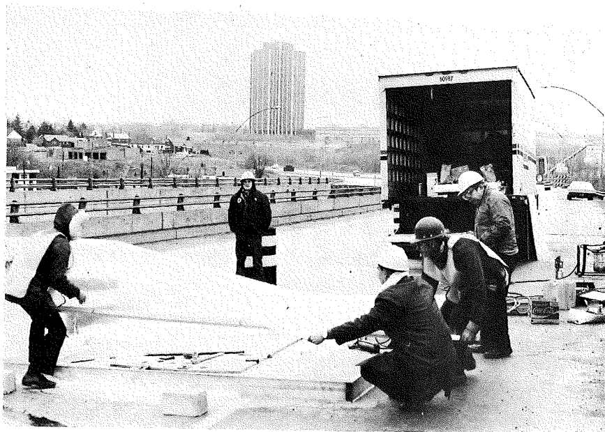
Fig. H-25 Covering of Working Area Against Rain
