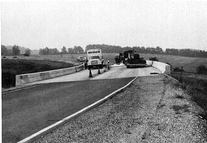
Fig. H-2 Close-Up View of PTI Test Track Bridge
