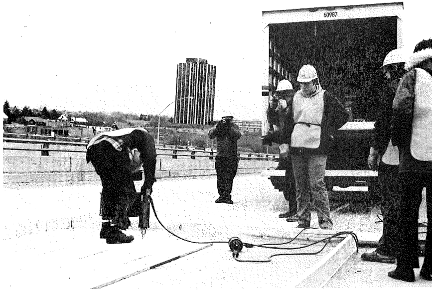
Fig. H-26 Drilling Bolt Holes for Impregnation Unit
