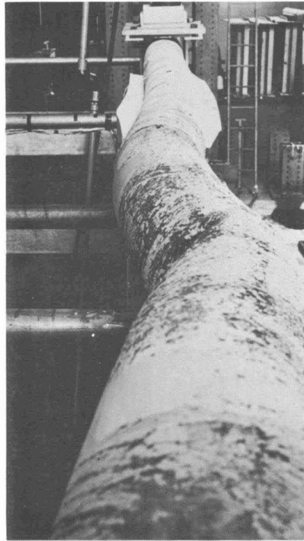
Fig. 2.37 Top Flange of Girder G5 after Testing
