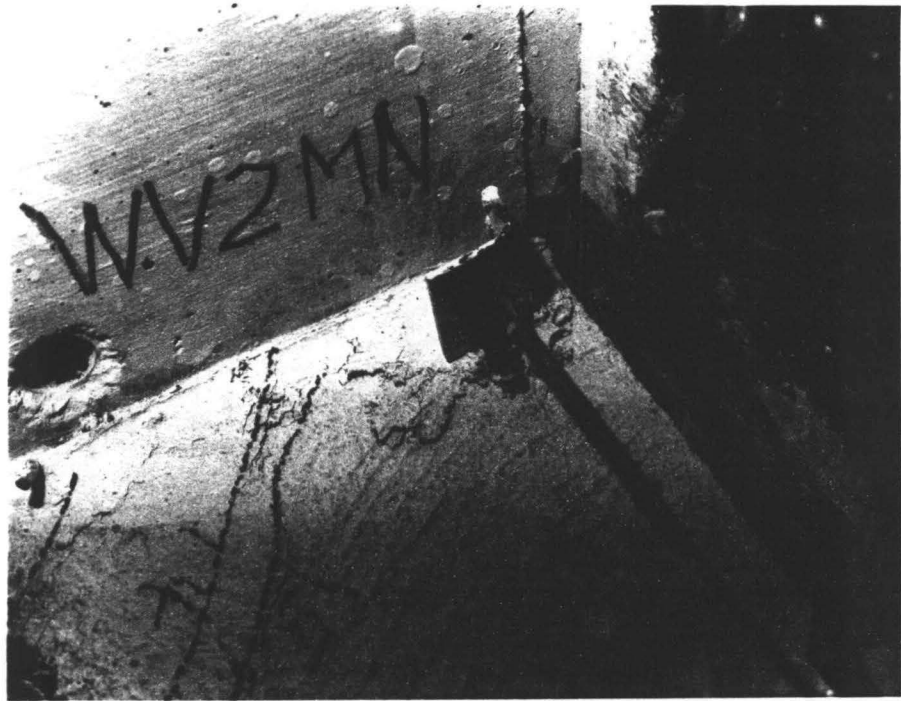
Fig 6.30 Concrete Crushing at the Compressive Corner
