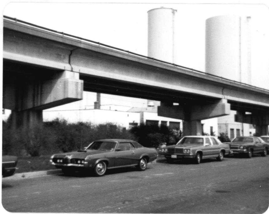
Fig. 17 One Complete Span of Collingswood Viaduct
