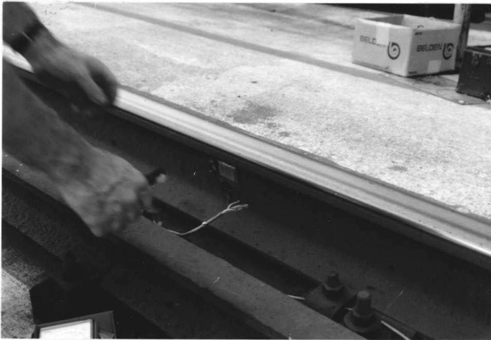
Fig. 6 Completed Installation of a Strain Gage to a Rail
