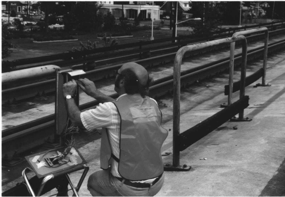
Fig. 8 Installation of Wiring to a Terminal Box
