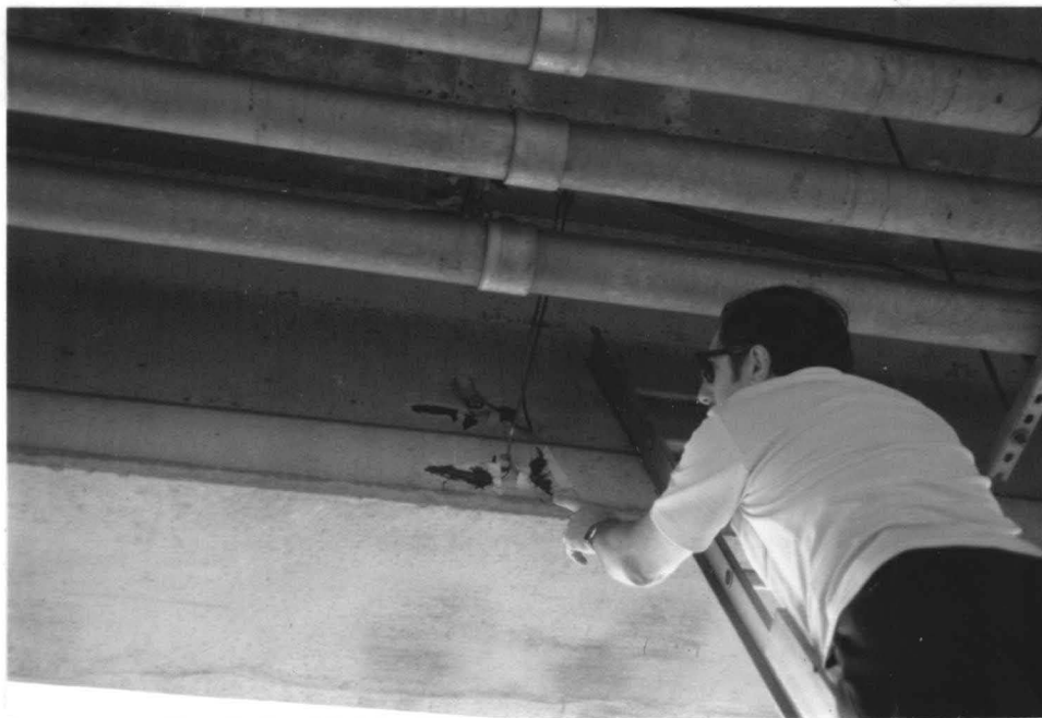
Fig. 7 Strain Gage Installation near the Bottom of a Prestressed Girder
