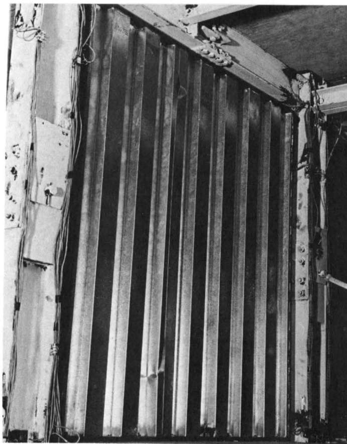
FIG. 51 DEFORMATION @ SEAM FASTENERS
