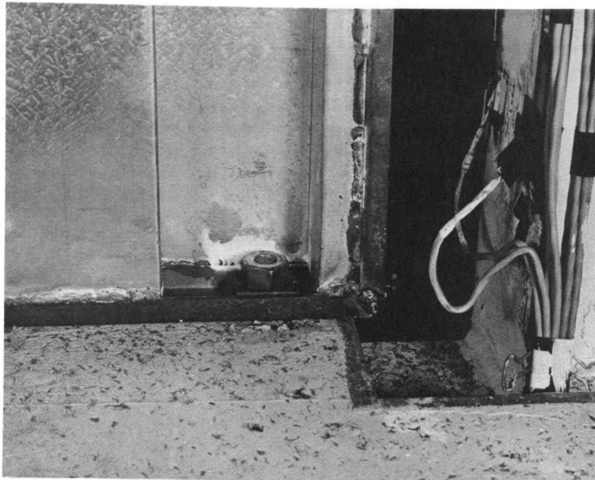
FIG. 19 PARTITION LOWER EDGE CONNECTION
